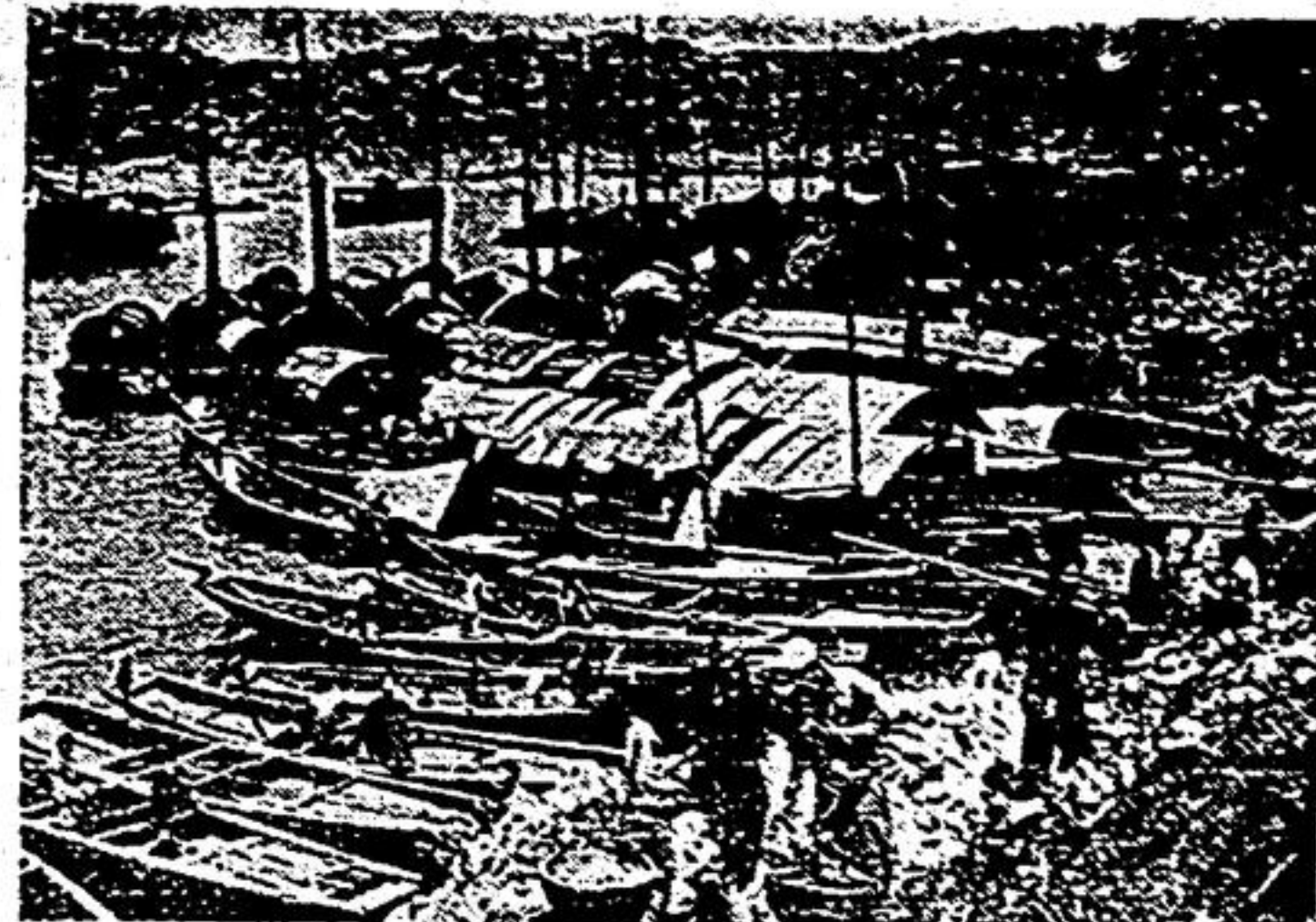
SAMPANS OVERTURN IN NANKING STORM — More than 130 persons were drowned at Nanking, China, when about 20 sampans, similar to those seen above, were overturned by the collapse of two floating pontoons and the bridge spanning them. Only 20 persons were rescued out of more than 150 who fell into the water. The pontoons were said to have collapsed following a sudden storm.
