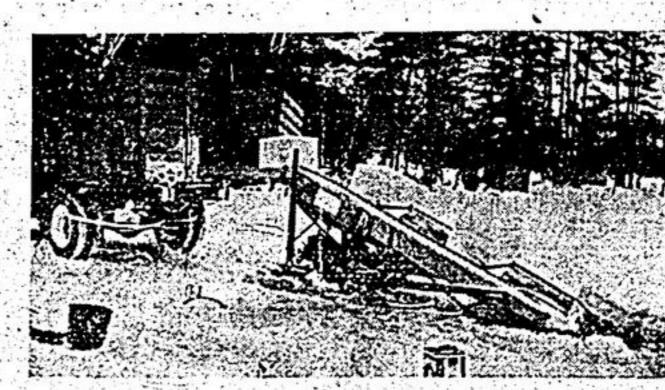
This is the loading device operated by Carl Rose which with ease hauled 12,500 cakes of ice out of the water up onto waiting
