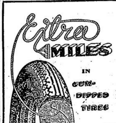
MUM-DIPPING which saturates every fibre and every strand of every cord with pure rubber, serves the same purpose as that of a cobbler waxing his thread . . . . prevents friction and multiplies strength.
