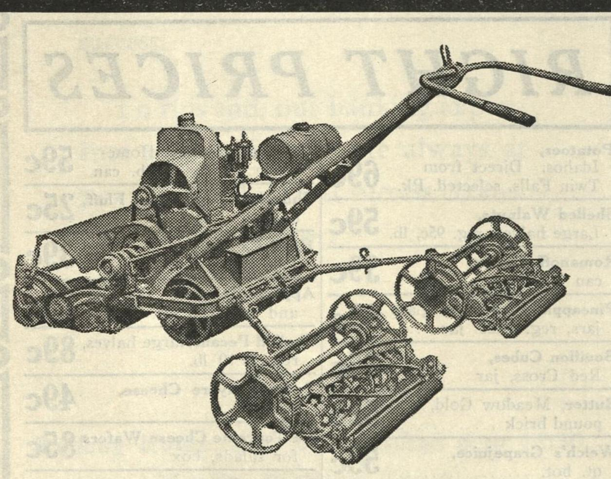
The Coldwell gasoline roller and mower has a cutting width, with attachment, of 60 inches. A good many Winnetka residents have found that they can save the cost of the machine the first season, with the added advantage of a better kept lawn.
