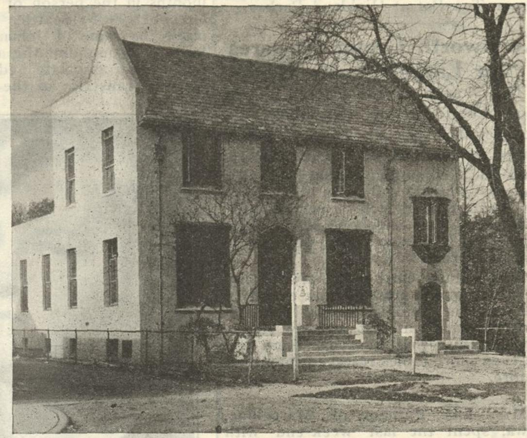
The original building was enlarged and remodeled to provide additional space for the operating and terminal rooms and operators' quarters. The north wall was taken out and the structure widened ten feet. Part of the rear wall was removed to permit a twenty-foot extension.
