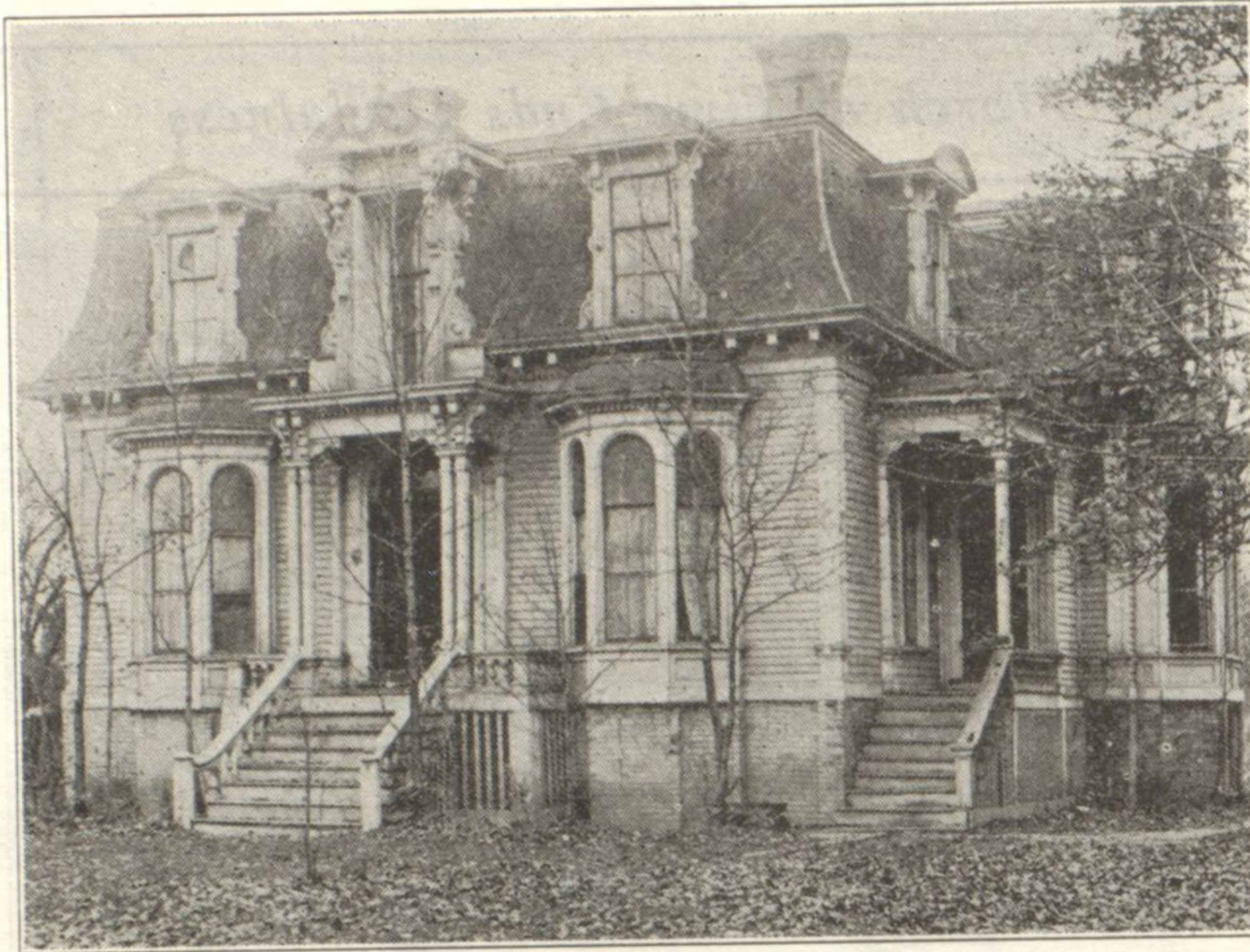
This once palatial residence, built by the late Dr. Alexander Hammond on Green Bay road, is to be torn down to make room for new homes.
