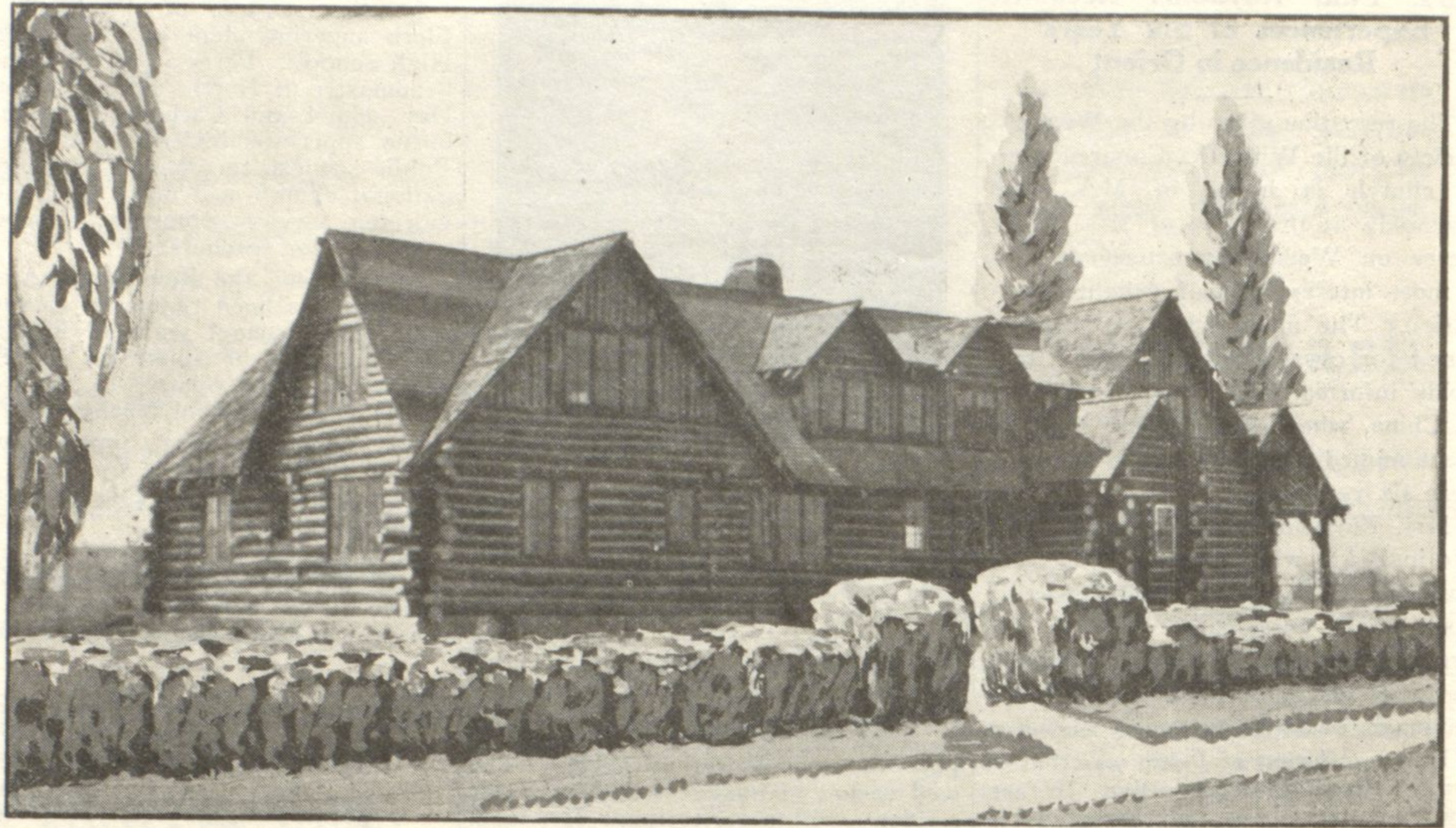
Here we have the uniquely designed administration building of the North Shore Military academy which is to open its door to cadets for the first time Monday, October 3. The architectural theme might readily suggest the old army post type of structure. The new school is located in Niles Center just south of the Evanston Golf club. An inaugural ball signaling the establishment of the new school is to be held in the Orrington hotel ballroom, Thursday, September 29.
