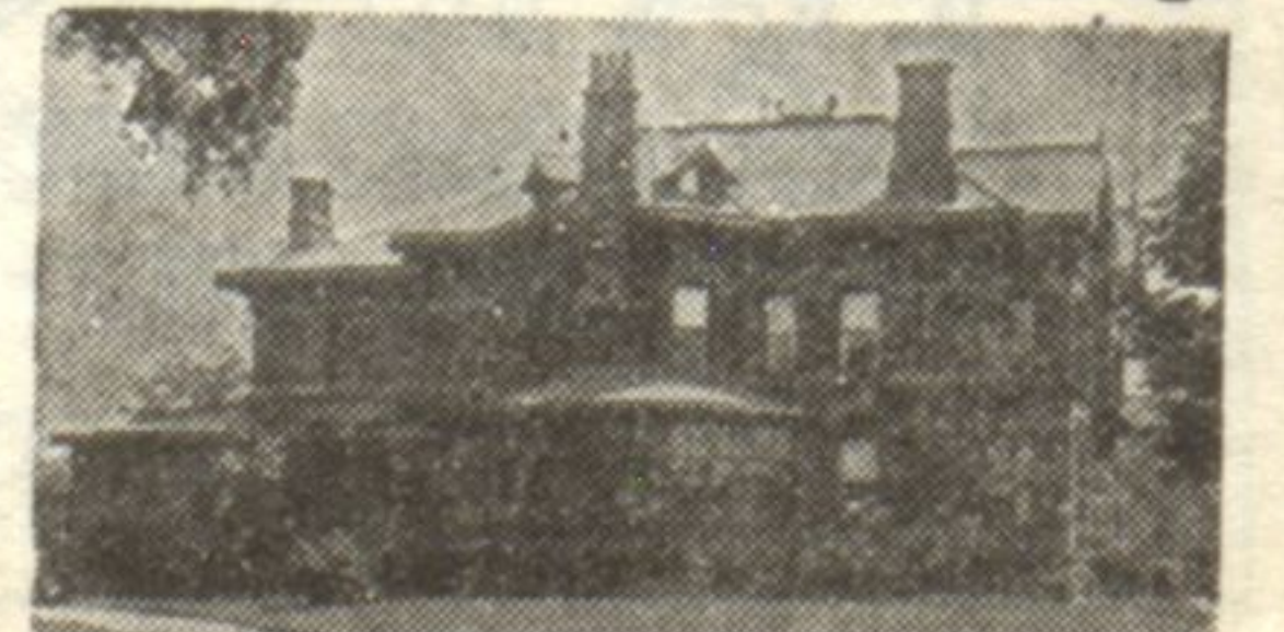
Students' Residence—in the heart of Chicago's finest residential district
