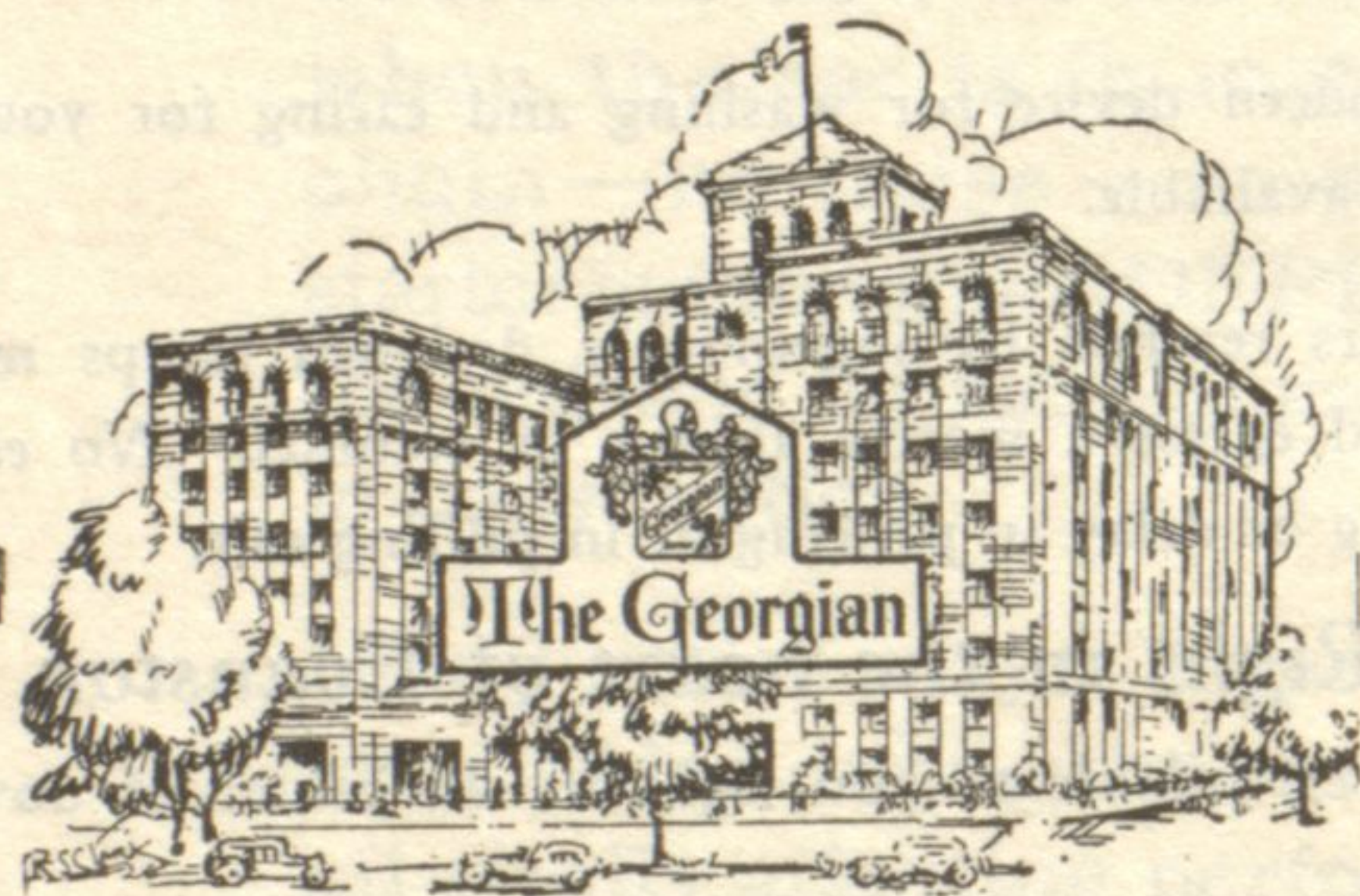
Hinman Avenue at Davis Street—Evanston
