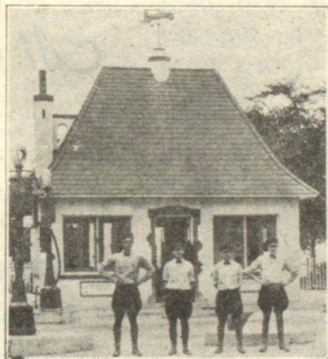
The Red Roof in No-Man's Land Just South of "The Cottage"
