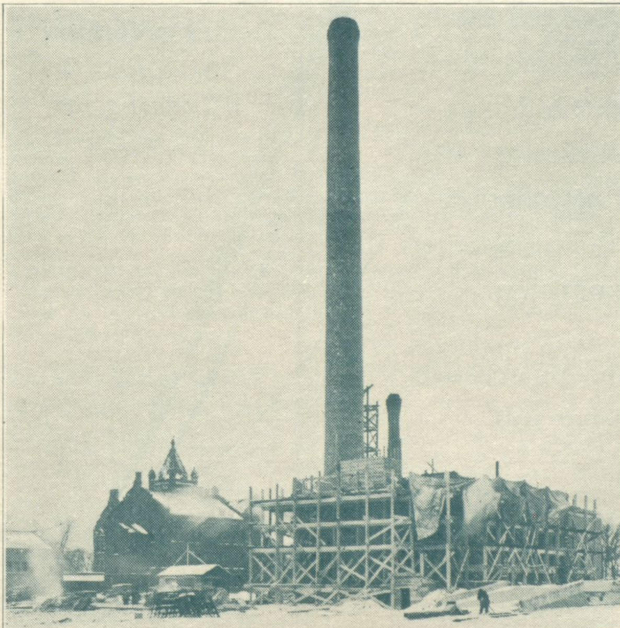
This is New Trier High school's new power plant, the first unit in the enlargement program of the school. The building will be completed within a month or six weeks, it is thought, and it will be put in operation next September. Modern oil burning equipment will be installed.
