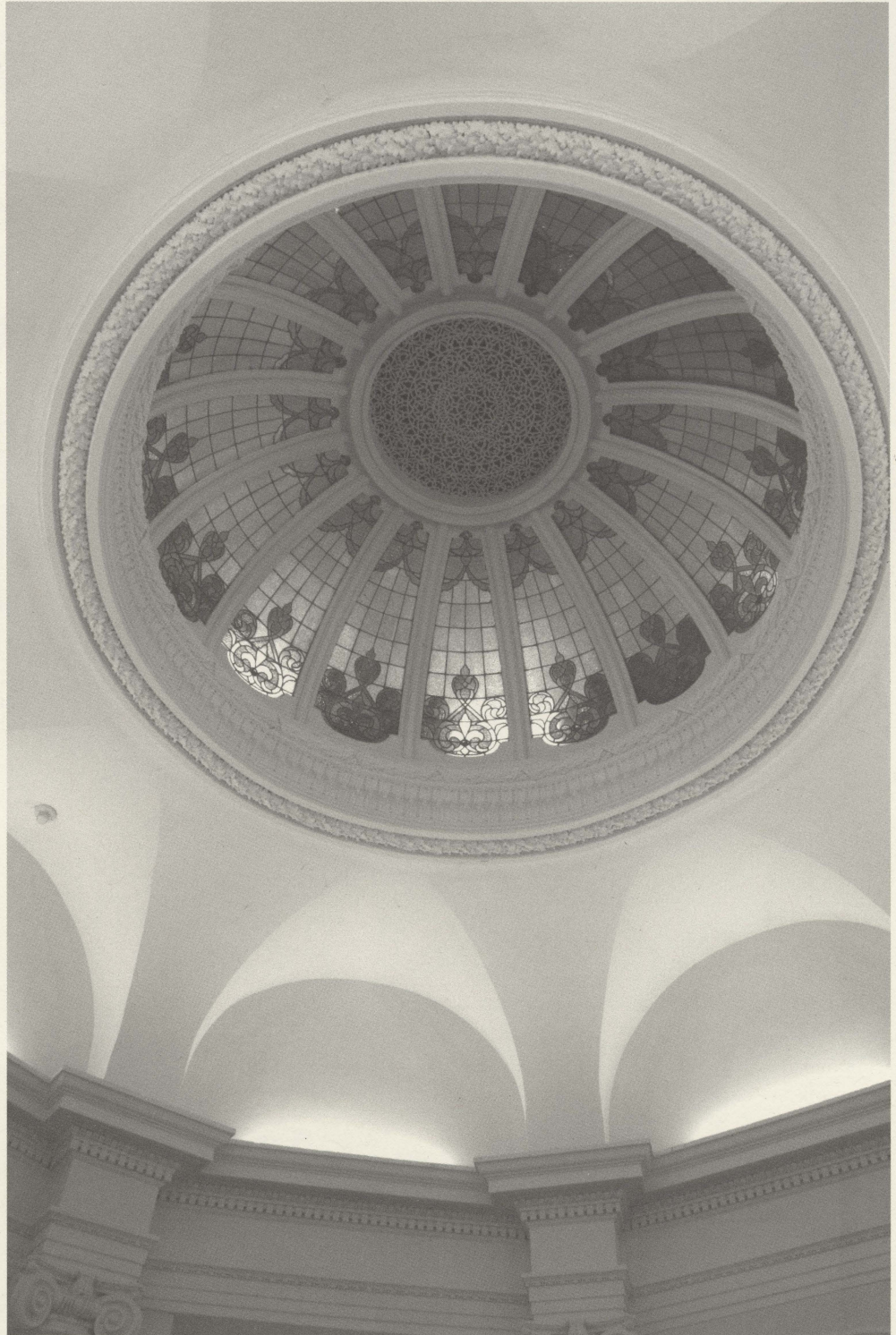
Carnegie Building, dome detail, Wilfrid Laurier University, Brantford, Ontario
