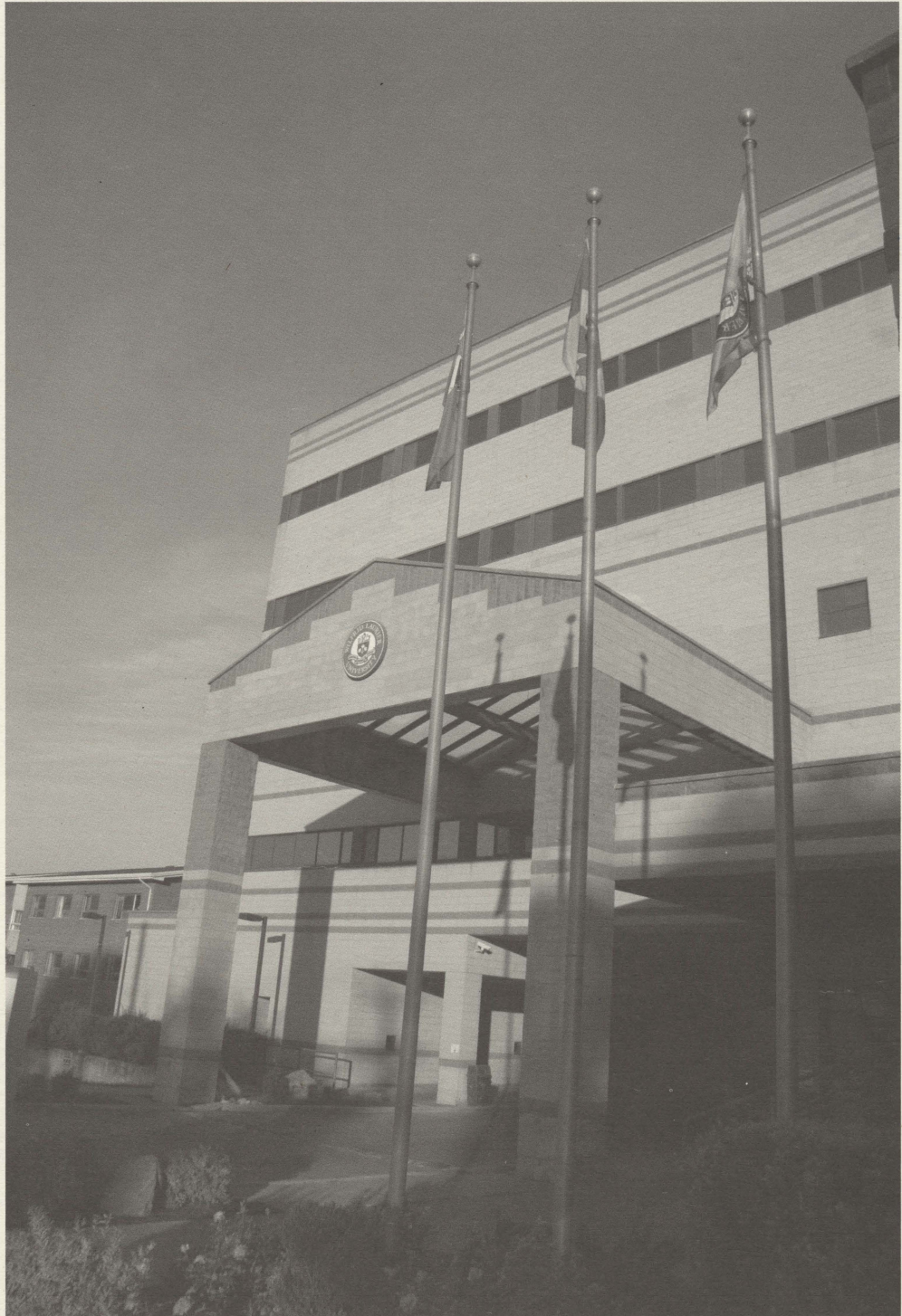
The Aird Building, Wilfrid Laurier University Campus, Waterloo, Ontario
