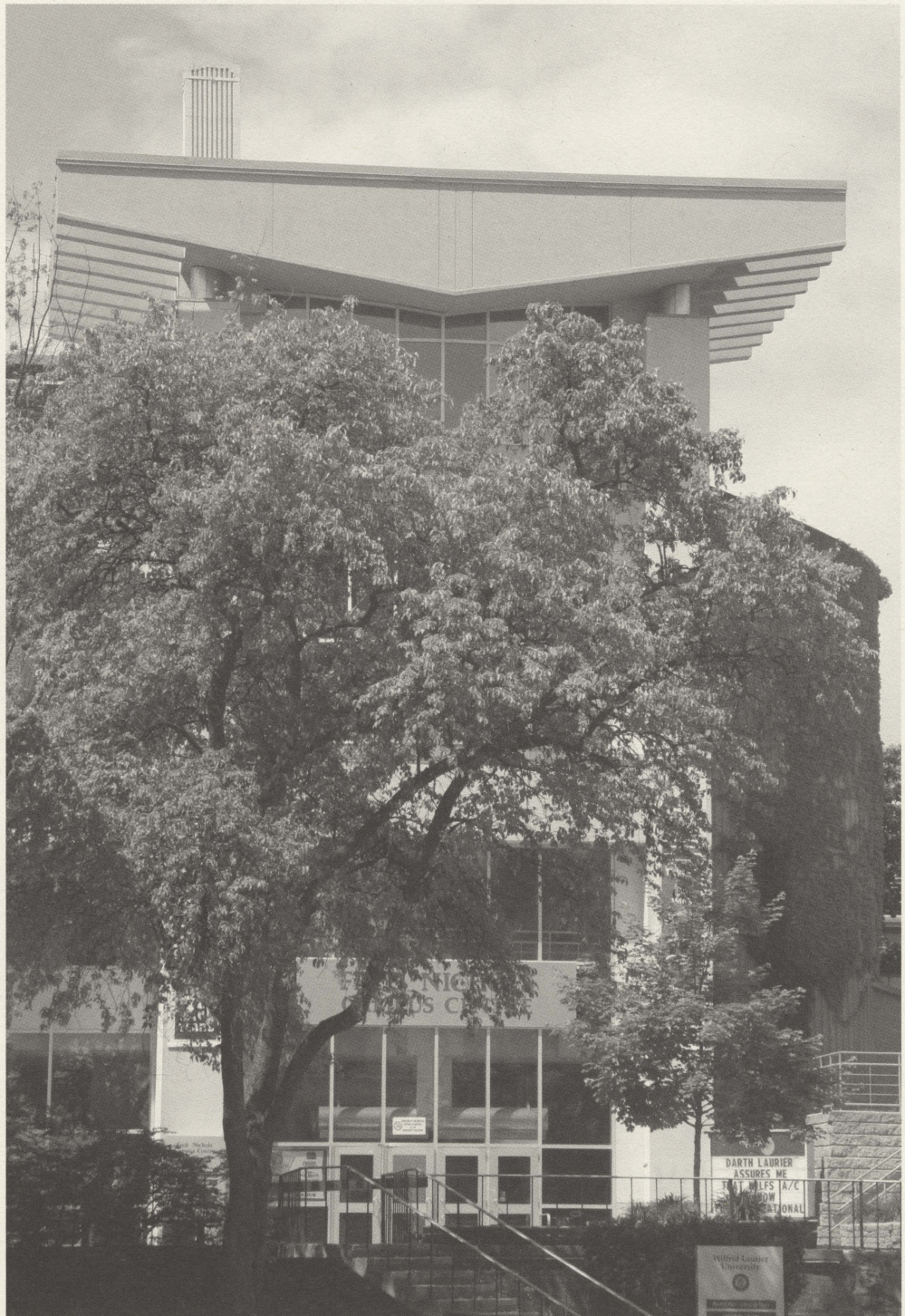
The Fred Nichols Campus Centre, Wilfrid Laurier University Campus, Waterloo, Ontario
