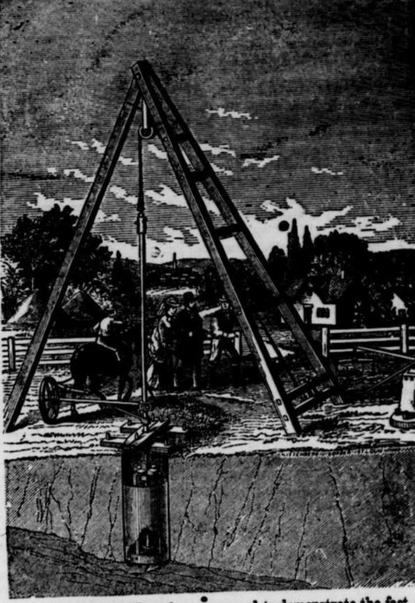
WE MEAN IT, and are prepared to demonstrate the fact. OUR AUGERS are operated entirely by HORSE POWER, and GUARANTEED to bore at the rate of 10 to 15 FEET PER HOUR.
