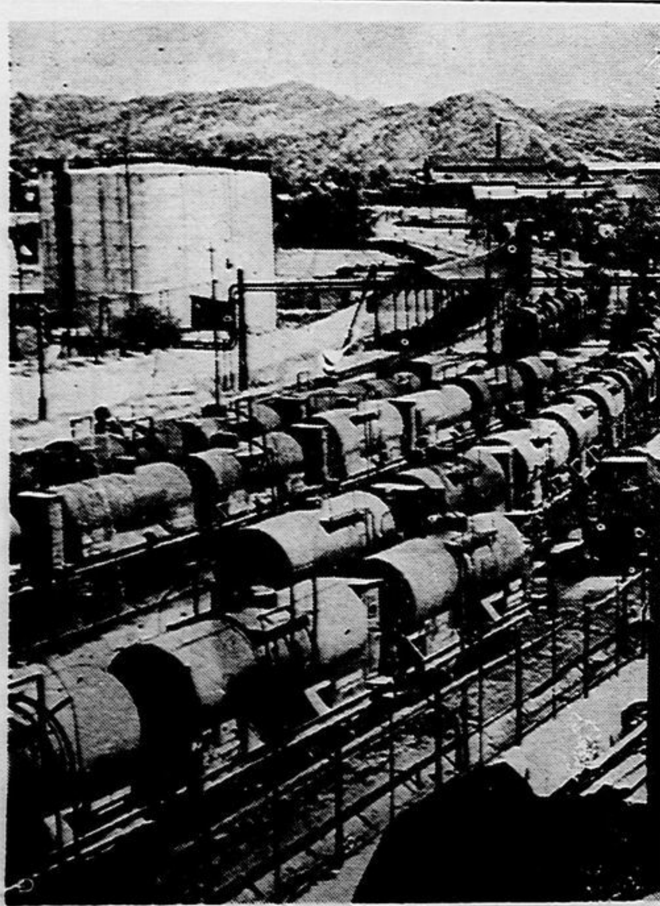
A view of a railway yard beside one of the many oil refineries in Rumania is seen above. The oil is piped down to the large tanks from the wells in the hills (background) and refined and pumped into the tank cars on the sidings. Rumania has ordered her already large military preparations speeded up, following authoritative reports that Germany was challenging the government's ban on export of aviation gasoline to the Reich.
