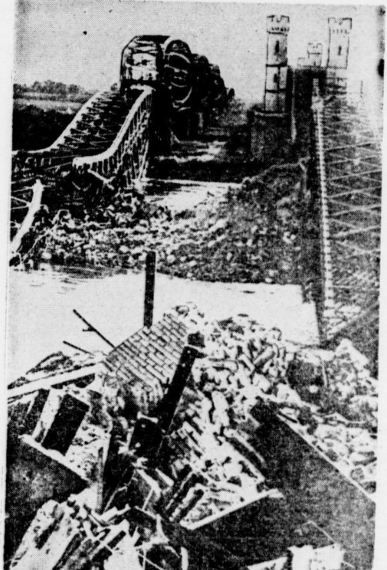
Retreating before the German advance, Polish army engineers wrecked this bridge over the River Weichsel at Dirschau in an effort to slow up German troop movements.
