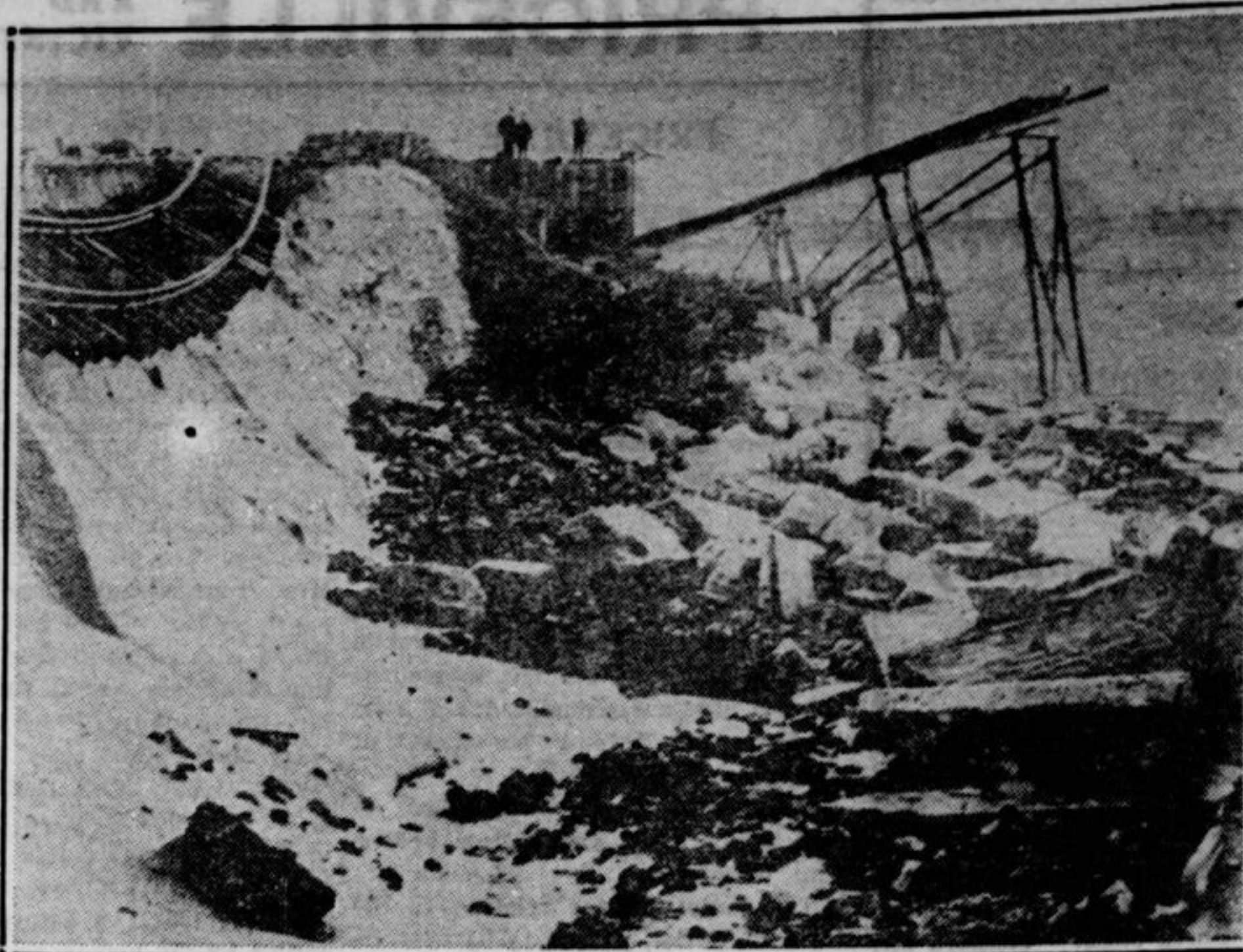
An angry sea pounded the shoreline of Borkum, Germany, leaving in its wake this scene of wreckage and demolition. This is typical of damage inflicted along the entire coast during the storm as wind-driven surf lashed seaboard.
