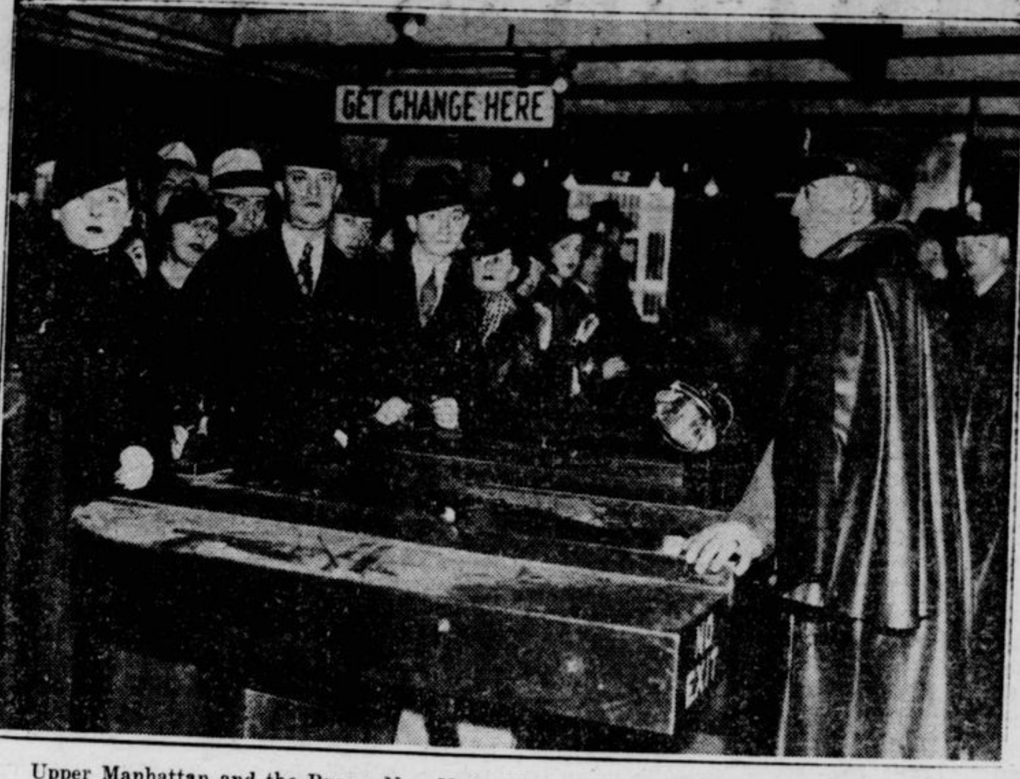
Upper Manhattan and the Bronx, New York City, were plunged into darkness and subway trains were stalled when power plant blast and fire paralyzed half the city's electrical system. Pictured is scene in subway station.
