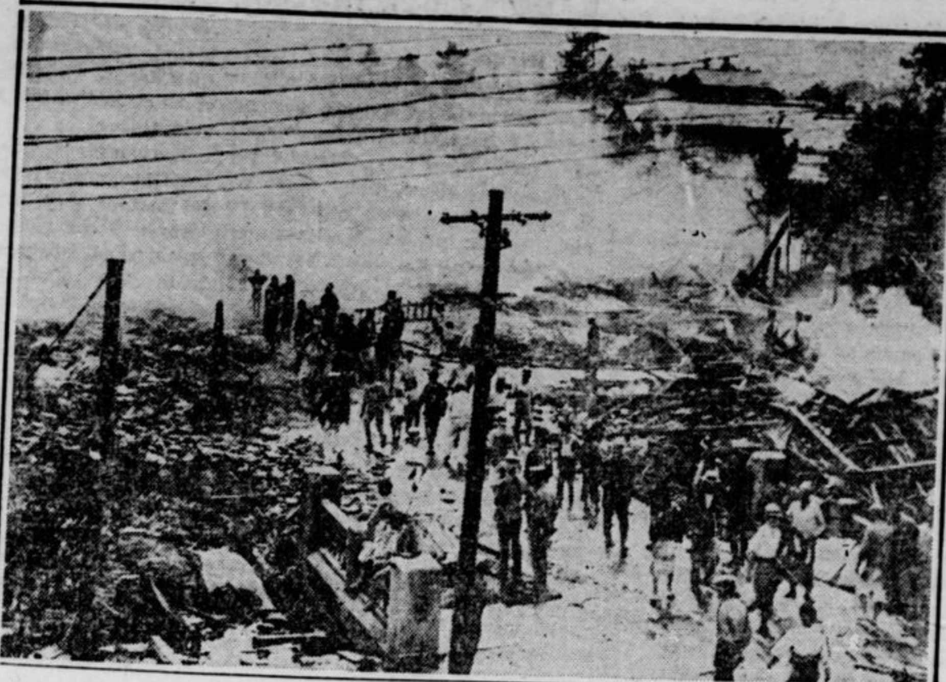
A general view of the desolation caused by fire that raged for six hours in the town of Shibata, Japan. The raging flames rendered 6,000 persons homeless and caused damage of more than $1,000,000.
