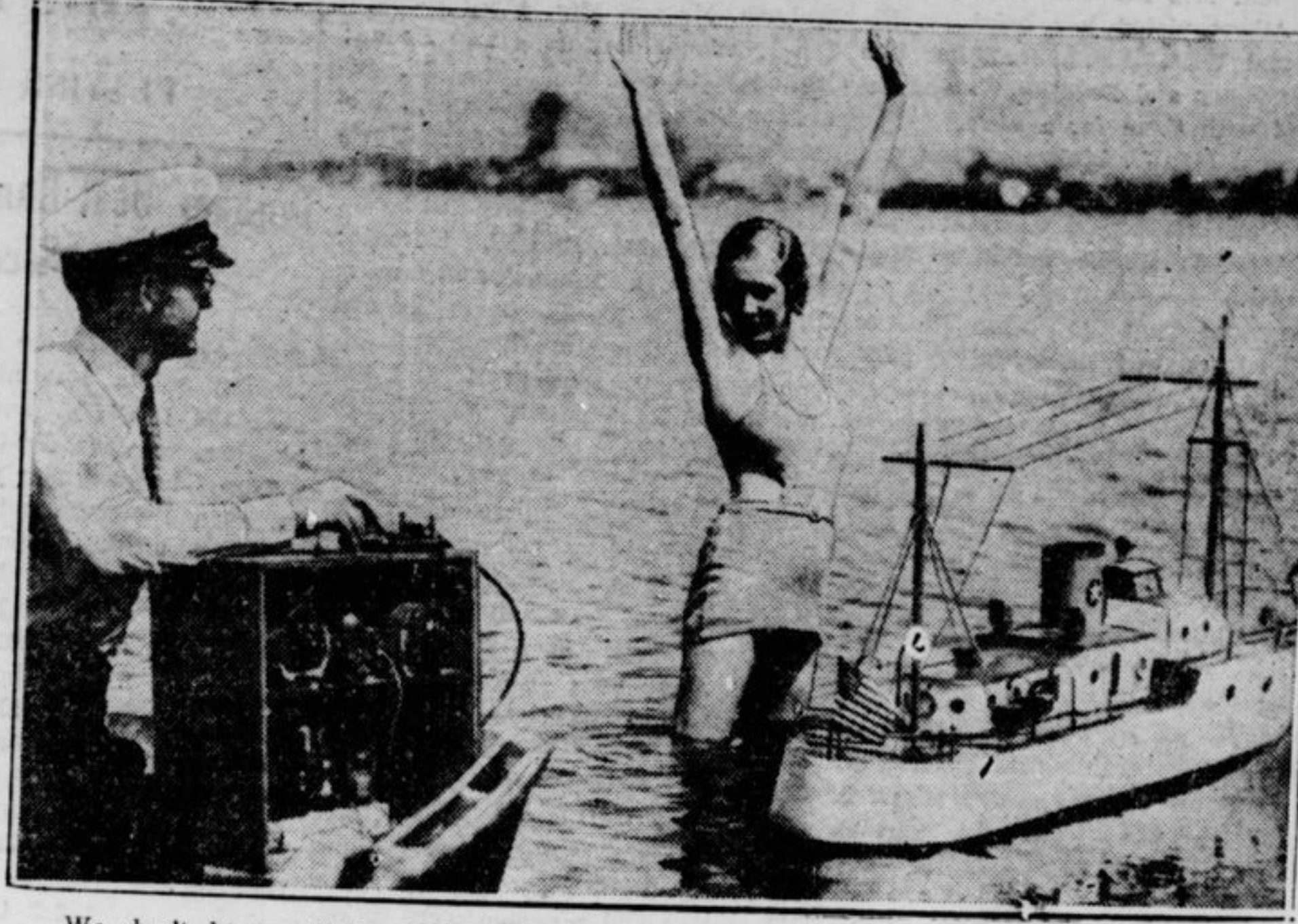
We don't know whether Miss Elsie Hobart is saying "Eureka" or just stretching from the fatiguing job of painting the miniature boat which Victor Carp started, stopped and steered entirely by radio control. The craft, 40 inches long, made a speed of two and a half knots during the demonstration.
