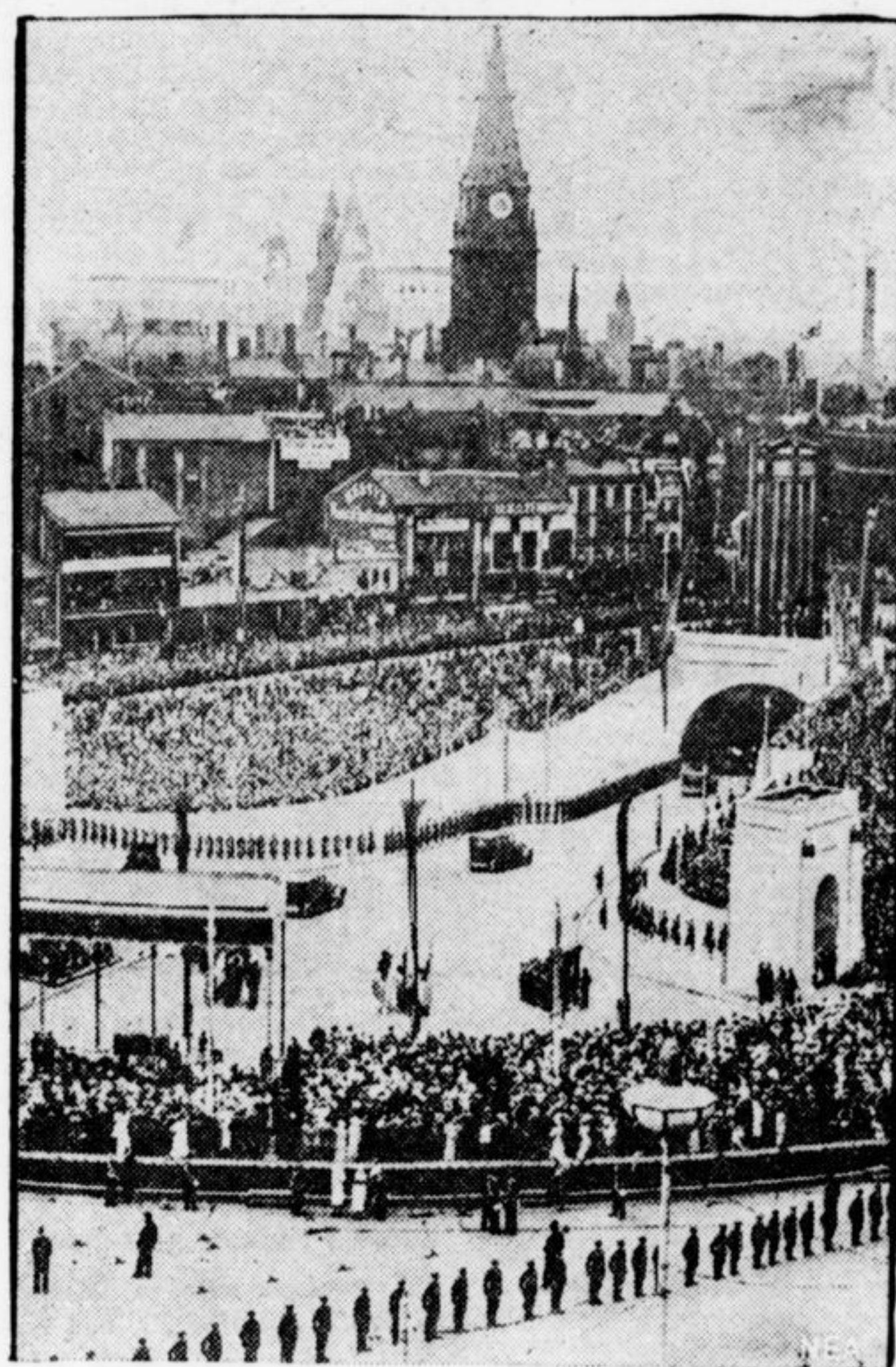
Part of the crowd of a million people, including hundreds of American vacationists, who gathered at Liverpool, England, for the formal opening by the King and Queen of the Mersey Tunnel, longest underwater tunnel in the world. Connecting Liverpool and Birkenhead, the tube is two miles long, took eight years to build and cost $40,000,000.
