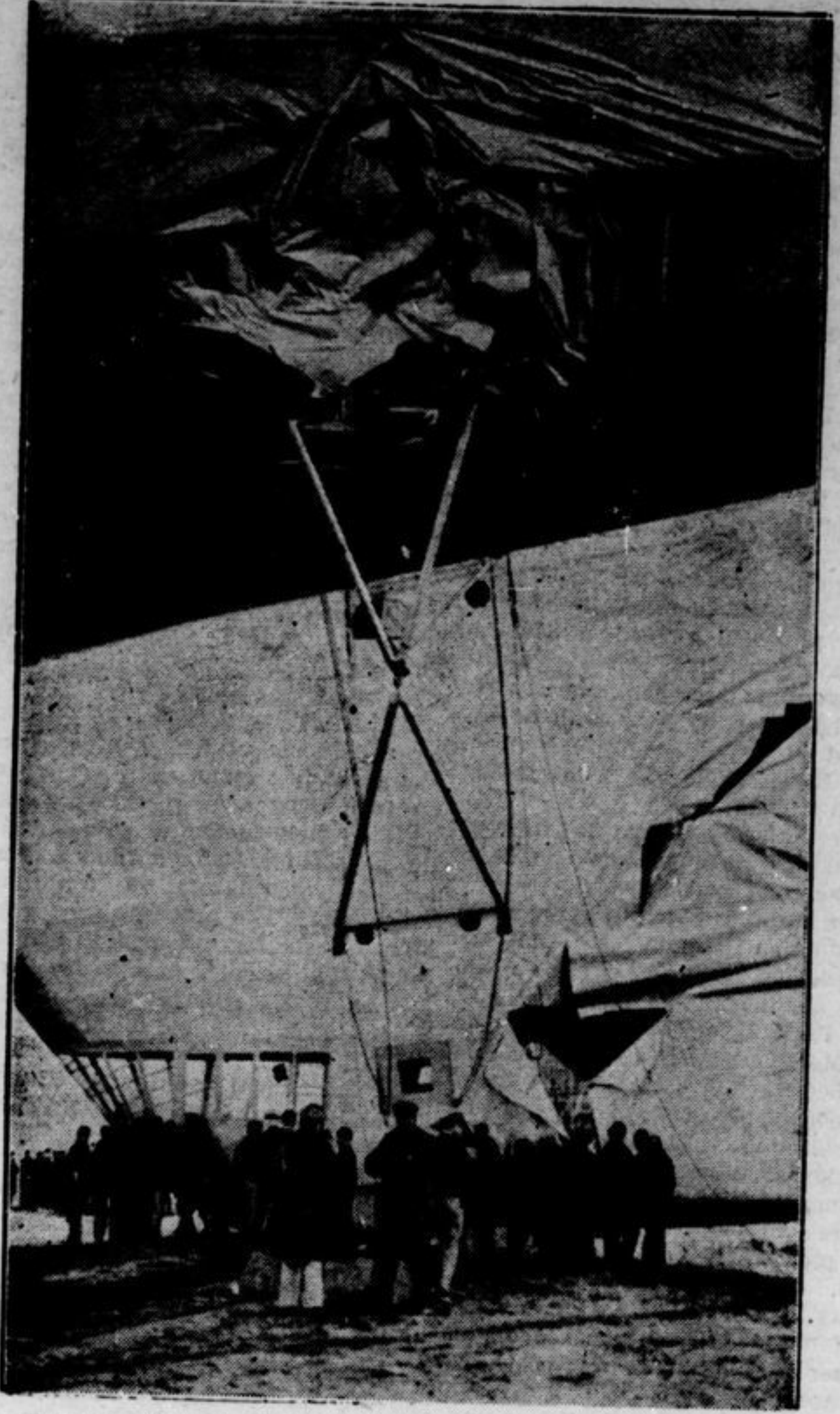
When a gust of wind bent the stern fin of the dirigible Akron to the ground the other day, two men were painfully injured, considerable damage done to the ship and five congressmen passengers got a fright.
