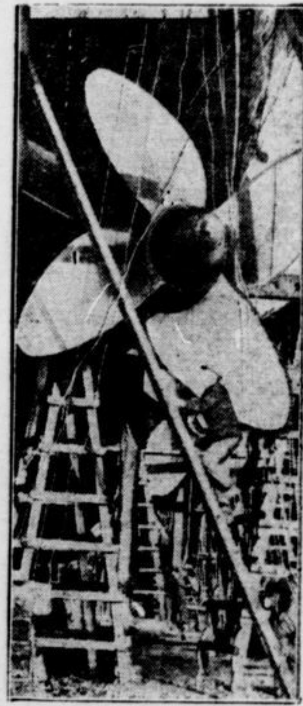
Here is the Aquitania at the Southampton floating dock, undergoing a thorough grooming in preparation for her next busy season. The propellers each weigh 15 tons.
