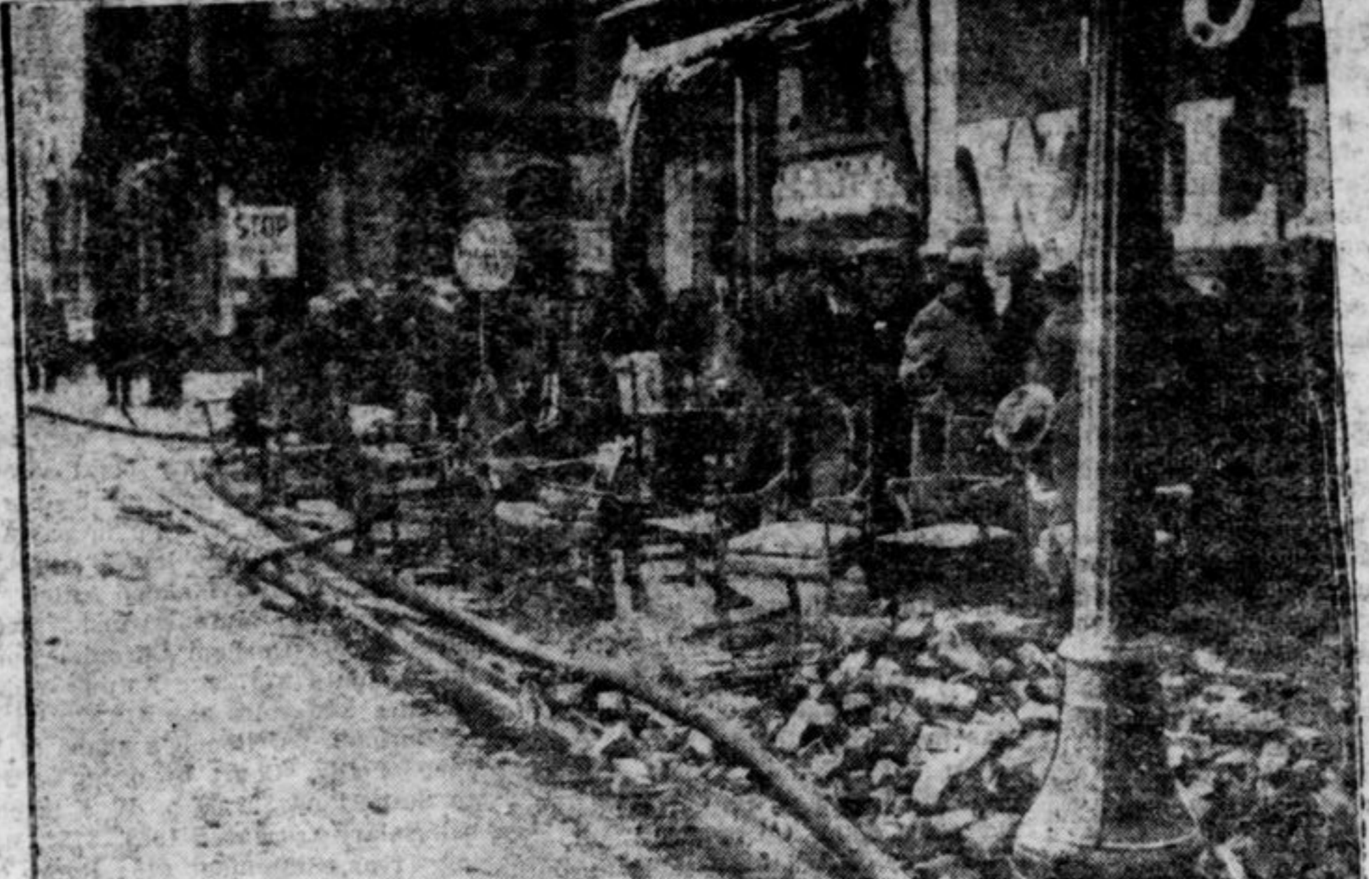
HALF-MILLION DOLLAR BLAZE SWEEPS CHATHAM All the furniture that was saved from the Garner Hotel, Chatham, after the fire of December 23, the worst in the history of the city.
