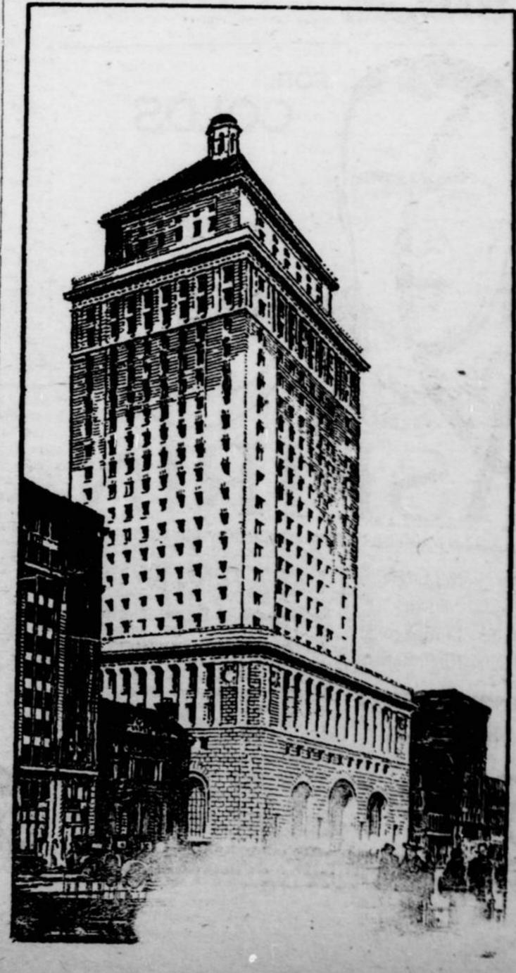
THE tallest office building, not only I in Canada, but in the British Empire, is at present under construction in Montreal. This building is the new Head Office of The Royal Bank of Canada. In its erection, Canadian materials are being used wherever possible. assive concrete foundations and retaining walls have been completed, and progress is rapidly being made on the steel superstructure, which is already showing above the surrounding fence.
