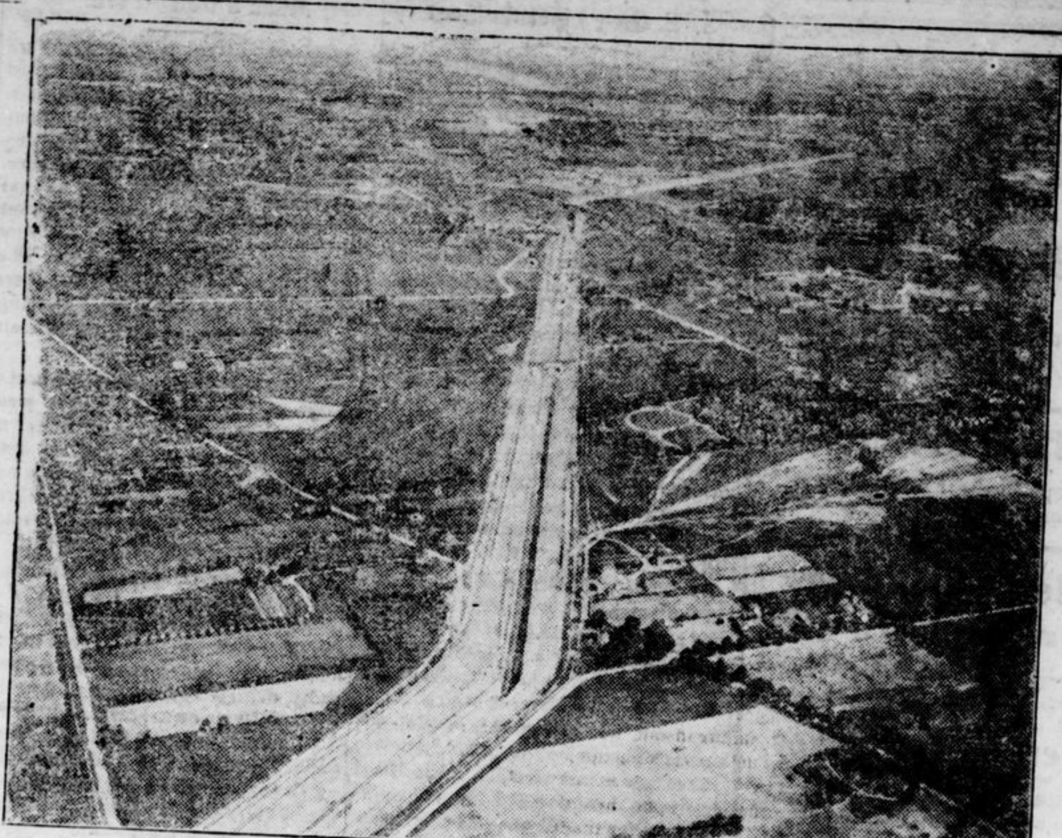
A BIRD'S-EYE VIEW OF THE CHIPPAWA POWER CANAL. In the distance can be seen the Niagara River, into which the canal discharges.
