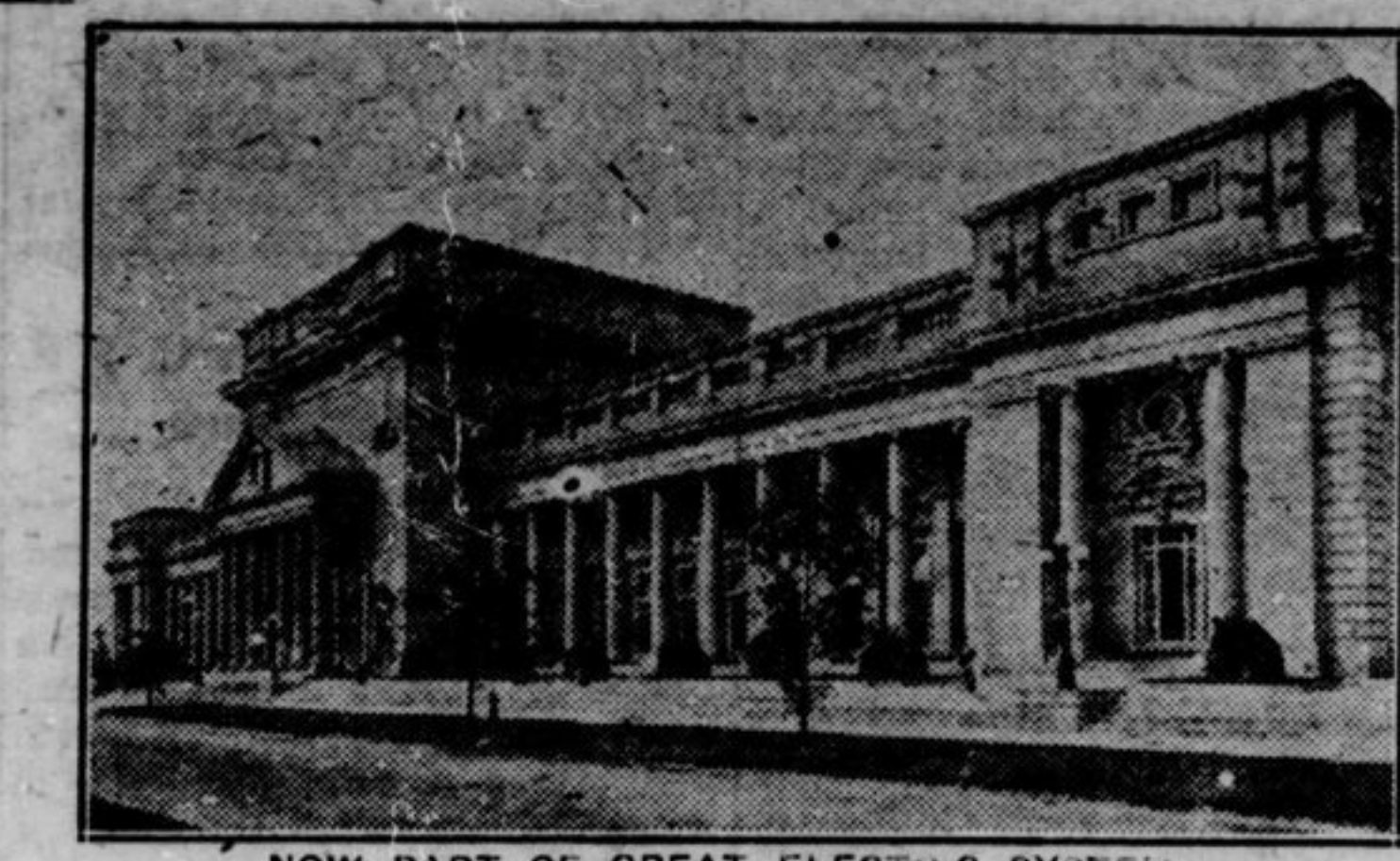
NOW PART OF GREAT ELECTRIC SYSTEM The Toronto Power House at Niagara Falls which becomes the property of the Ontario Hydro-Electric Commission under the recent purchase of the McKenzie interests.
