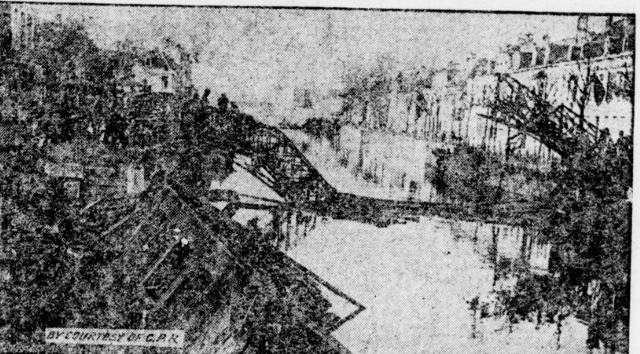
The River Scheldt and broken bridge at Tournal.
