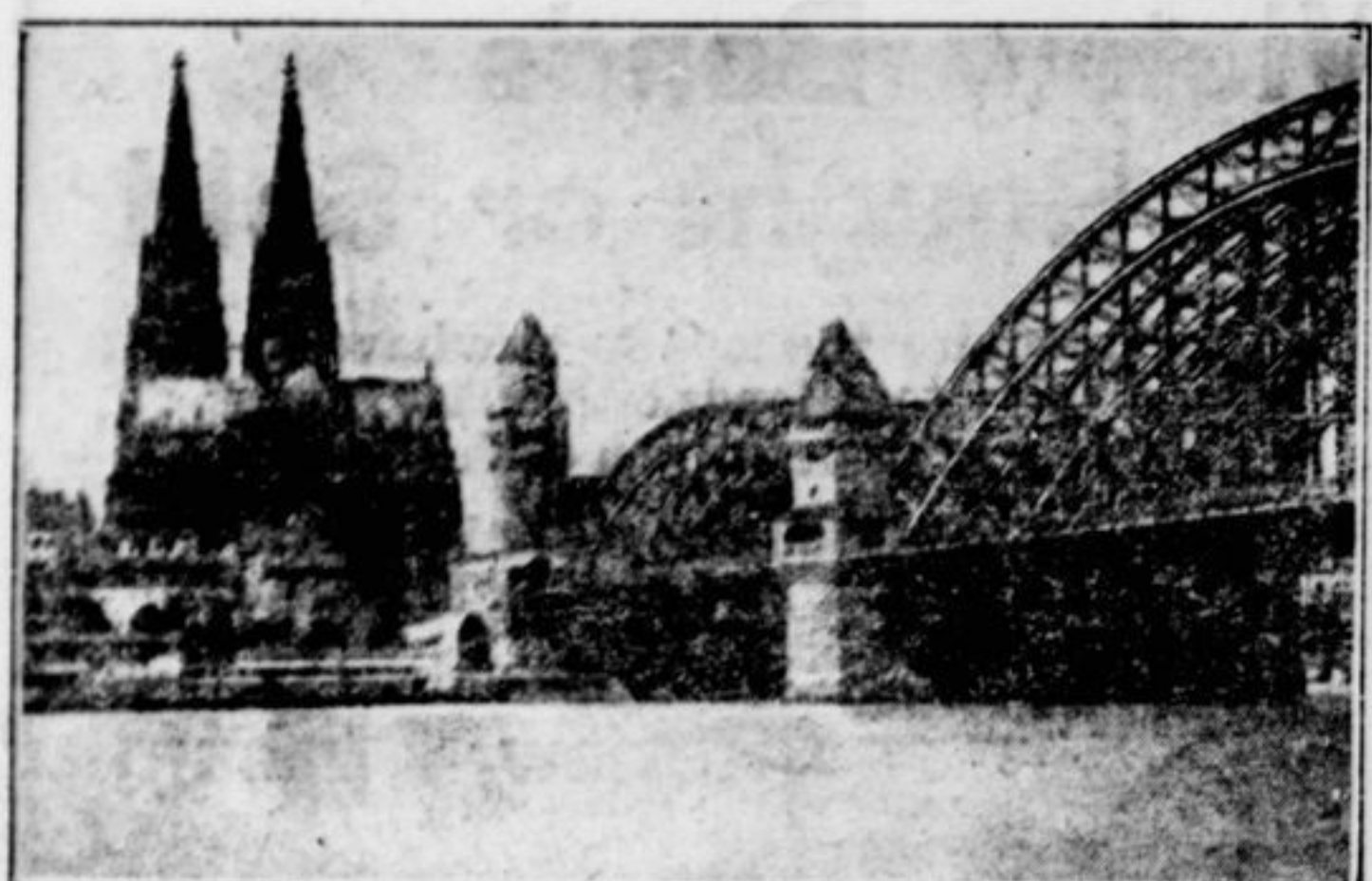
A section of the large bridge across the Rhine at Cologne, known as the Hohenzollern bridge. In his letter accompanying, C. C. Ramage says 'our 1st Division marched across in full battle strength, taking seven hours to cross the bridge.' In the distance is seen the famous Cologne Cathedral.
