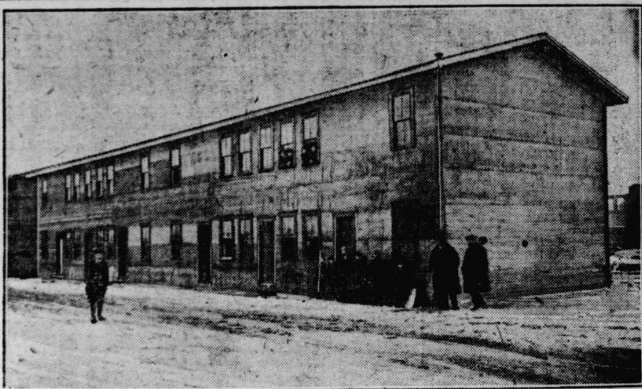
One of the quickly constructed huts in Halifax, which has housing capacity for six separate families.
