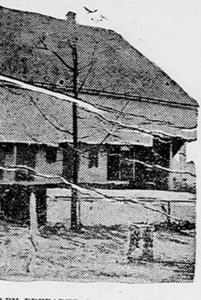
BARN PREPARED FOR FUMIGATION.
