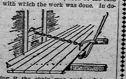
ing it the chain was anchored to window sill or studding. The handle of the cant hook was placed against a flooring board and the hook caught into a link of the chain. The handle was then pulled back, forcing the flooring boards into place. When doing this a block should be placed between the hook on the chain and the window. sill and also between the cant hook handle and the flooring :- Correspondent of Missouri Valley Farmer.
