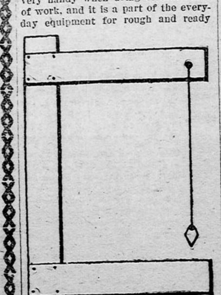
farm carpentering and building. The one illustrated here is easy to make. Very little material is required. Take two ordinary laths, get them set true with the try-square or T-square and attach the bob with a string. By using the illustration as a guide you can make a very serviceable help.-Farm
