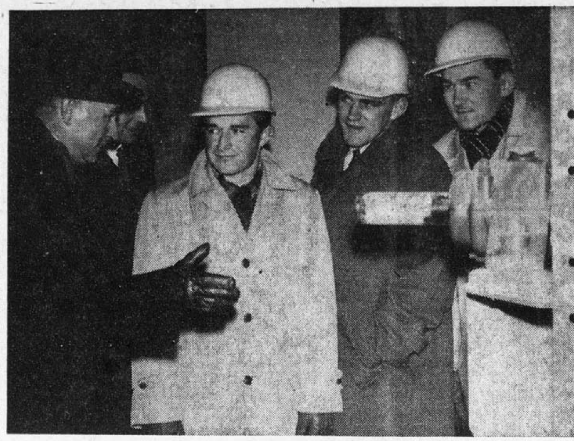
Examining one of the air-conditioning units in the new multi-million dollar Union Carbide building in Toronto are three third-year students from the School of Architecture, University of Toronto, during a recent field trip. H. Cannon (left), building maintenance supervisor, UCC Ltd., and A. Brighton, representative of Shore and Moffat, project architects, explain the operation of the unit, left to right: J. I. Kalhok, Simcoe; D. N. Wilson, Guelph, and A. F. Jammer, Hampton.
