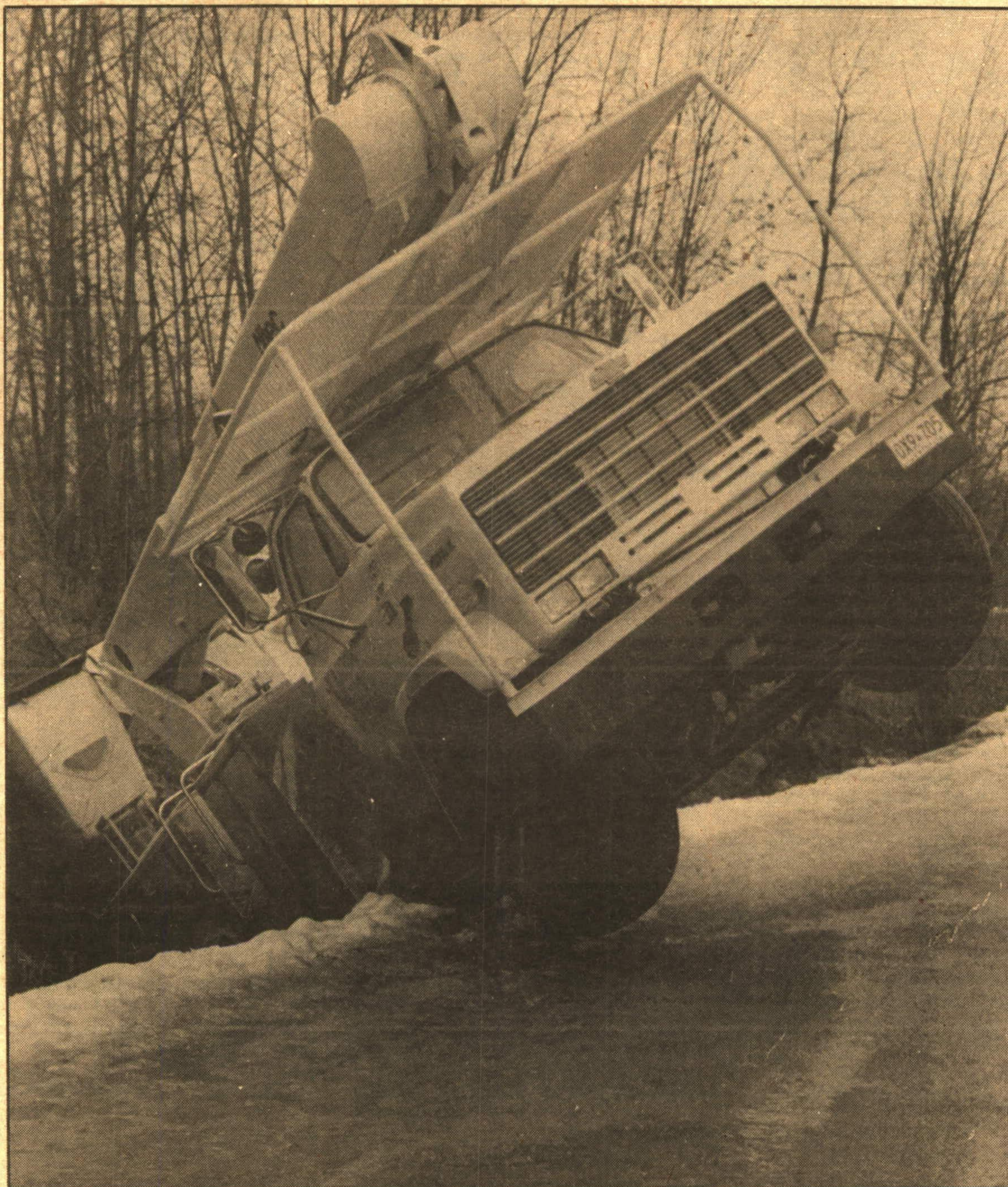
Whoops! This Halton Hills Hydro truck found Thursday morning's ice storm made roads around the utility's construction project in Acton treacherous. The rear end of the truck slid down the embankment into the School Creek lifting the
