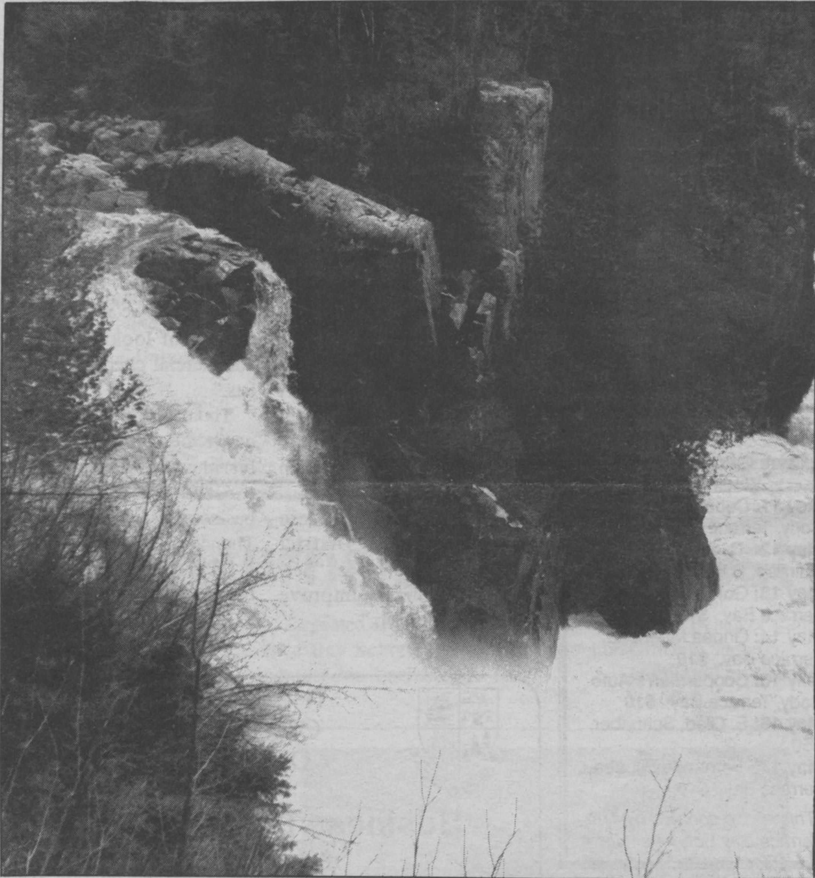
Ontario Hydro opened the Aguasabon River dam last week, giving this impressive view of the gorge from the newly built observation deck.
