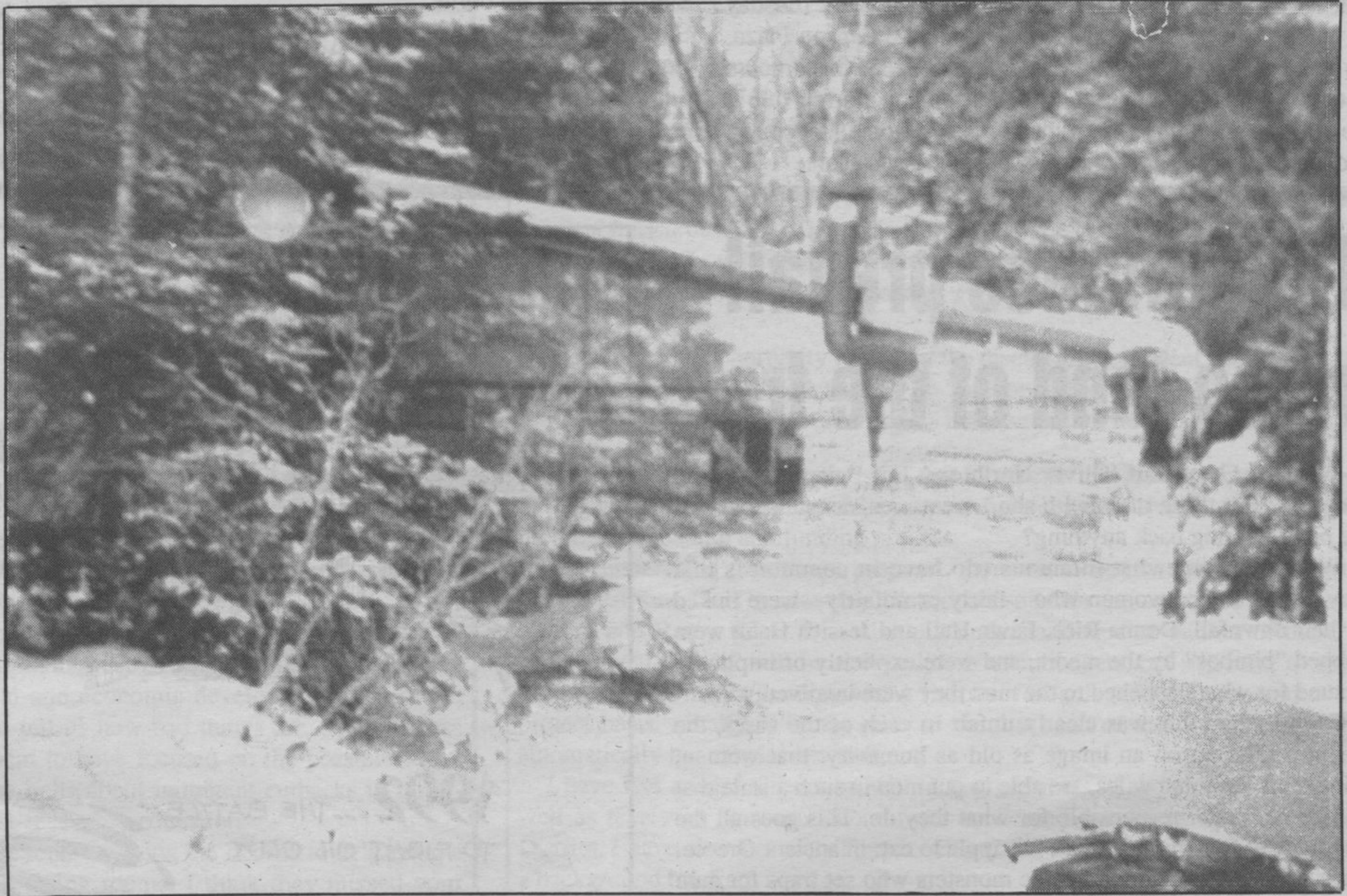
Illegal cabins, like the one pictured above, are becoming more and more common, says the MNR's Ken McWatters. "People are getting better at building them, and they're getting better at hiding them," he says.
