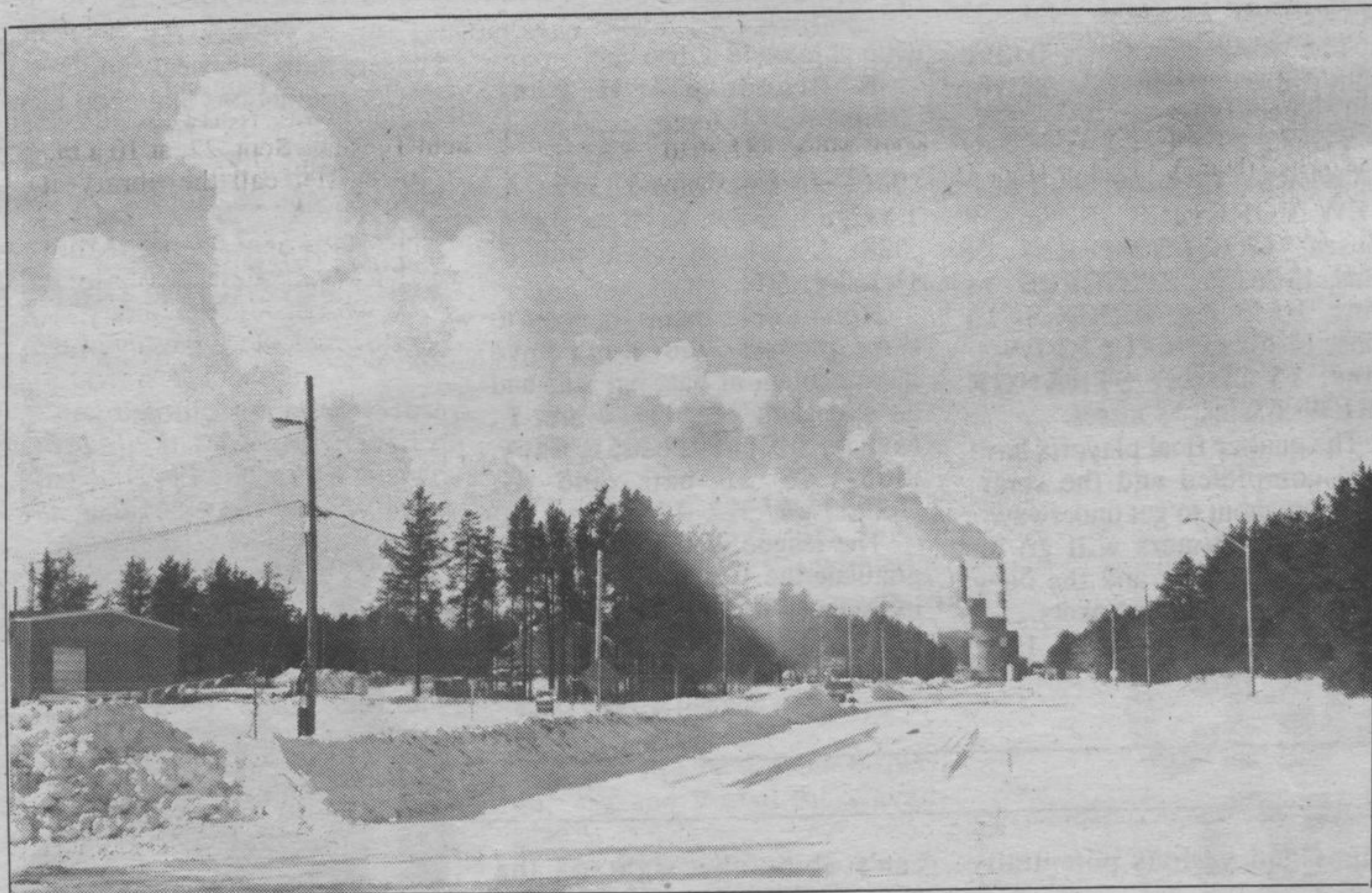
The Kimberly-Clark pulp mill in Terrace Bay, Ontario.
