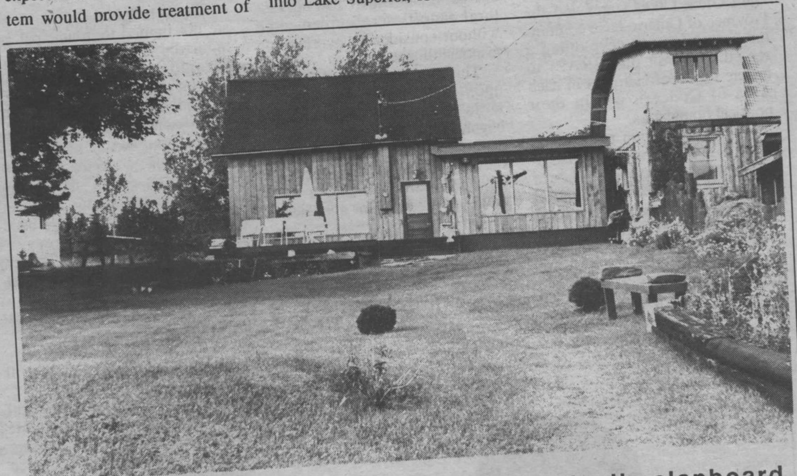
This house was built in 1884. It was originally clapboard.
