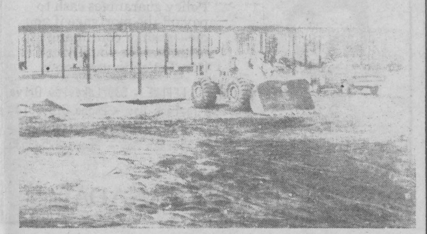
Pictured here is the new McCausland Hospital in its present stage of construction. The floor and roof are expected to be completed within two weeks. Workers are now busy with welding and applying the aluminum finish. Although the carpenters' strike this summer slowed down operations, construction has since accelerated rapidly and is now on schedule.
