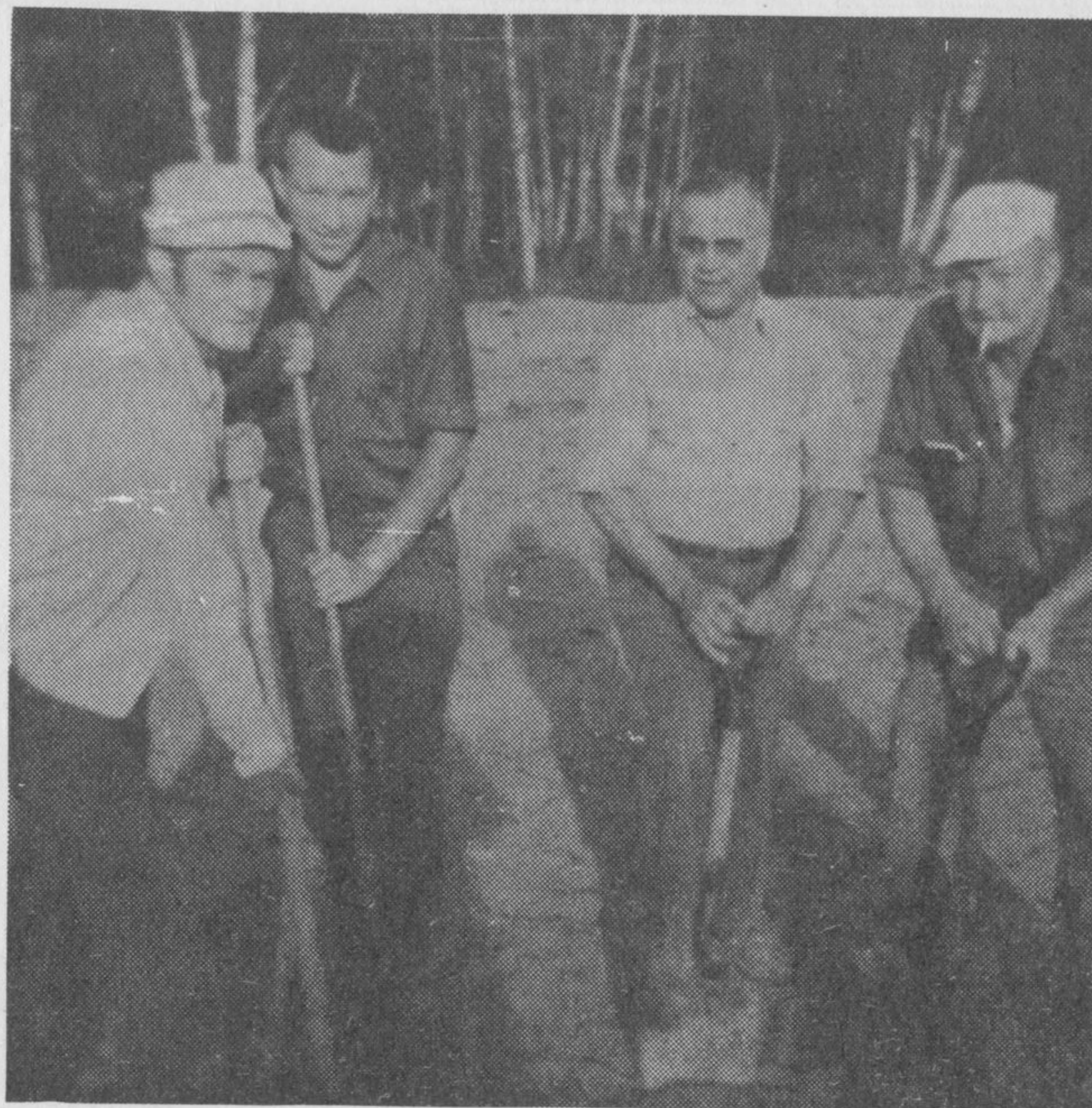
The site for the new Legion building on Highway 17, near Fort Garry Road, has been cleared and levelled.
