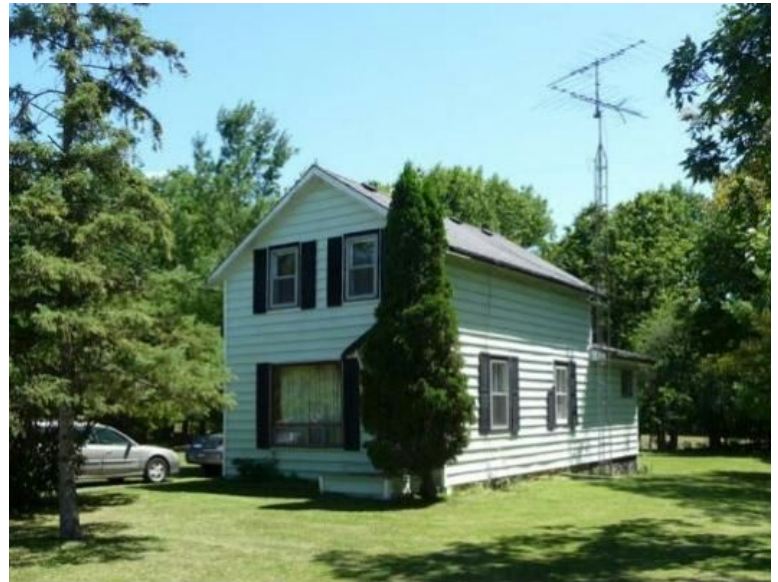
3388 Burnhamthorpe Road West, photo taken by Heritage Oakville
