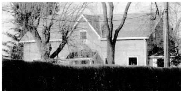
3269 Dundas Street West (North Side, W of Bronte)
