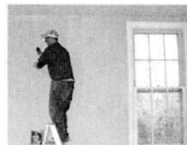
Jamie preparing the wall
