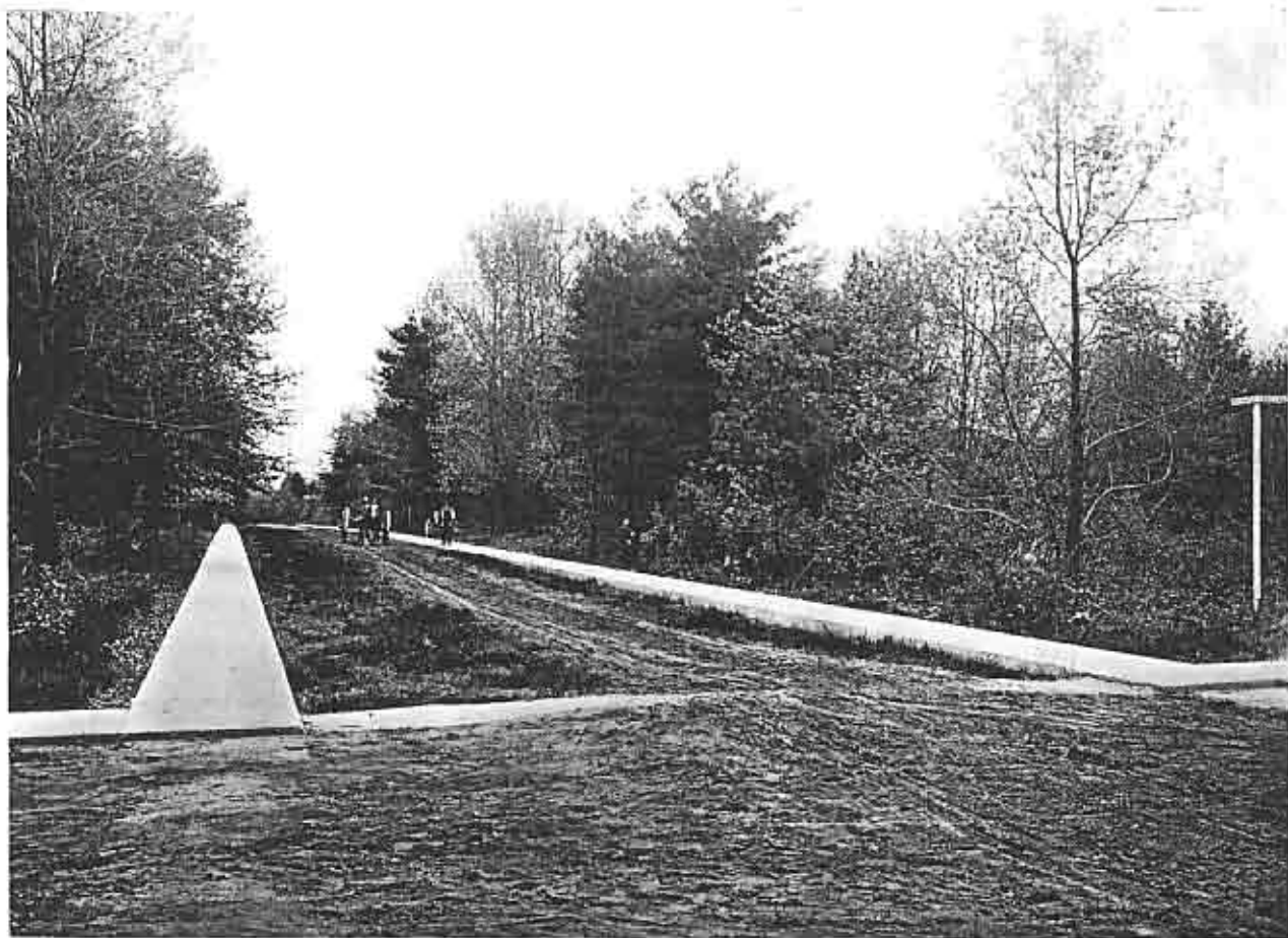
Watson Avenue, Brantwood, looking North. Corner of Galt Ave.
