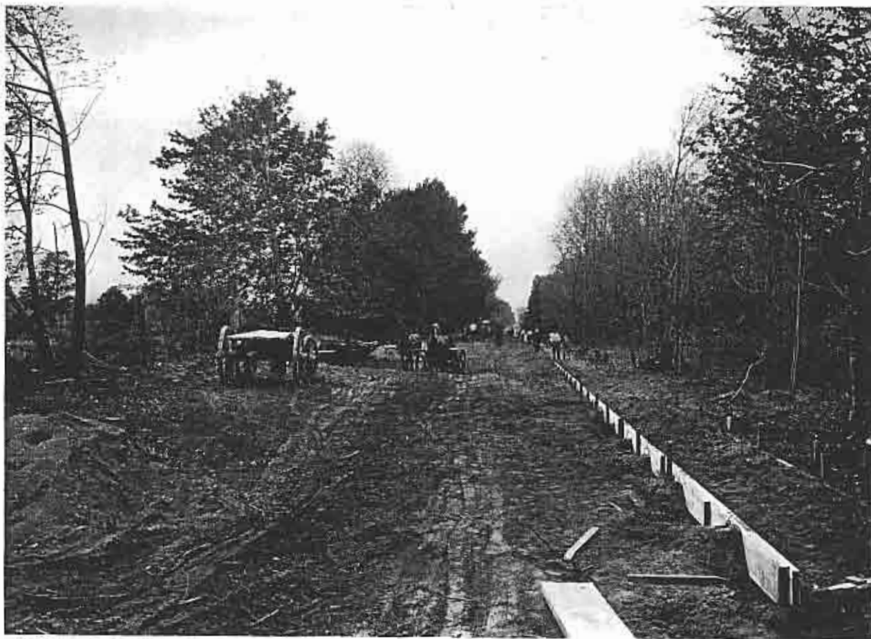
Grading on Gloucester Road, Brantwood.
