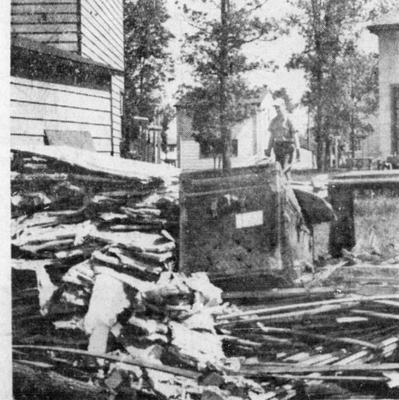
Tons of plaster and wood are being carted out of Winnipeg homes as citizens concentrate on repairing flood damage. Water destroyed walls and foundations as well as flooring and furniture. This pile of wallboard, plaster, furniture and miscellaneous household equipment came from one house, that of George Gilmour in the Wildwood Park area.
