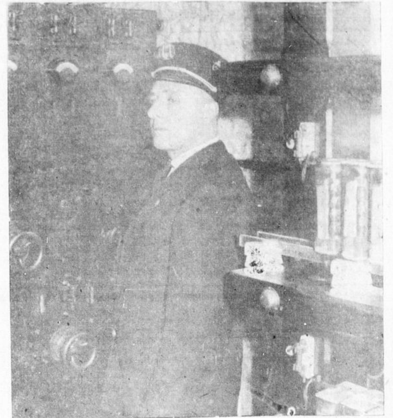
DEPARTMENT GENERATES OWN POWER: Captain Gordon Pooley, supervisor of the local fire alarm system, stands at the control board in the big battery room as he prepares to make the twice-daily check-up of the system. At his right is one of the banks of batteries which provide "juice" for the system. The department has its own power supply, as the risk in break-downs in the public power service is too great.
