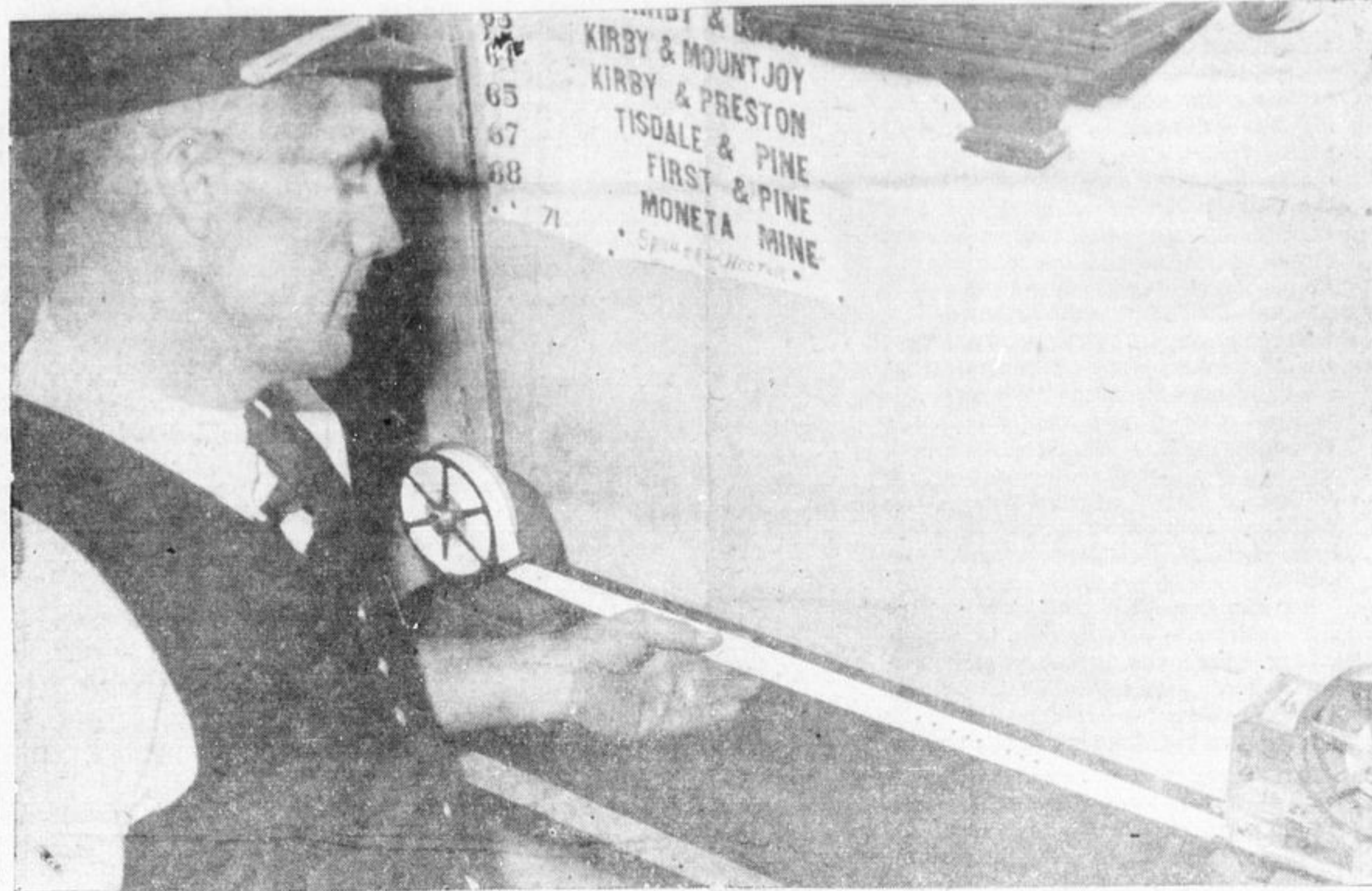
HOW ALARMS ARE LOCATED: Lieutenant Frank Culhane of the Timmins fire department here examines the moving tape installed at the front of the local fire hall. This tape, controlled electrically, registers the location of fire boxes from which fire alarms are put in. Note the two groups of perforations on the tape, one a group of five and one of three. This indicates that an alarm has been rung on box number 53.
