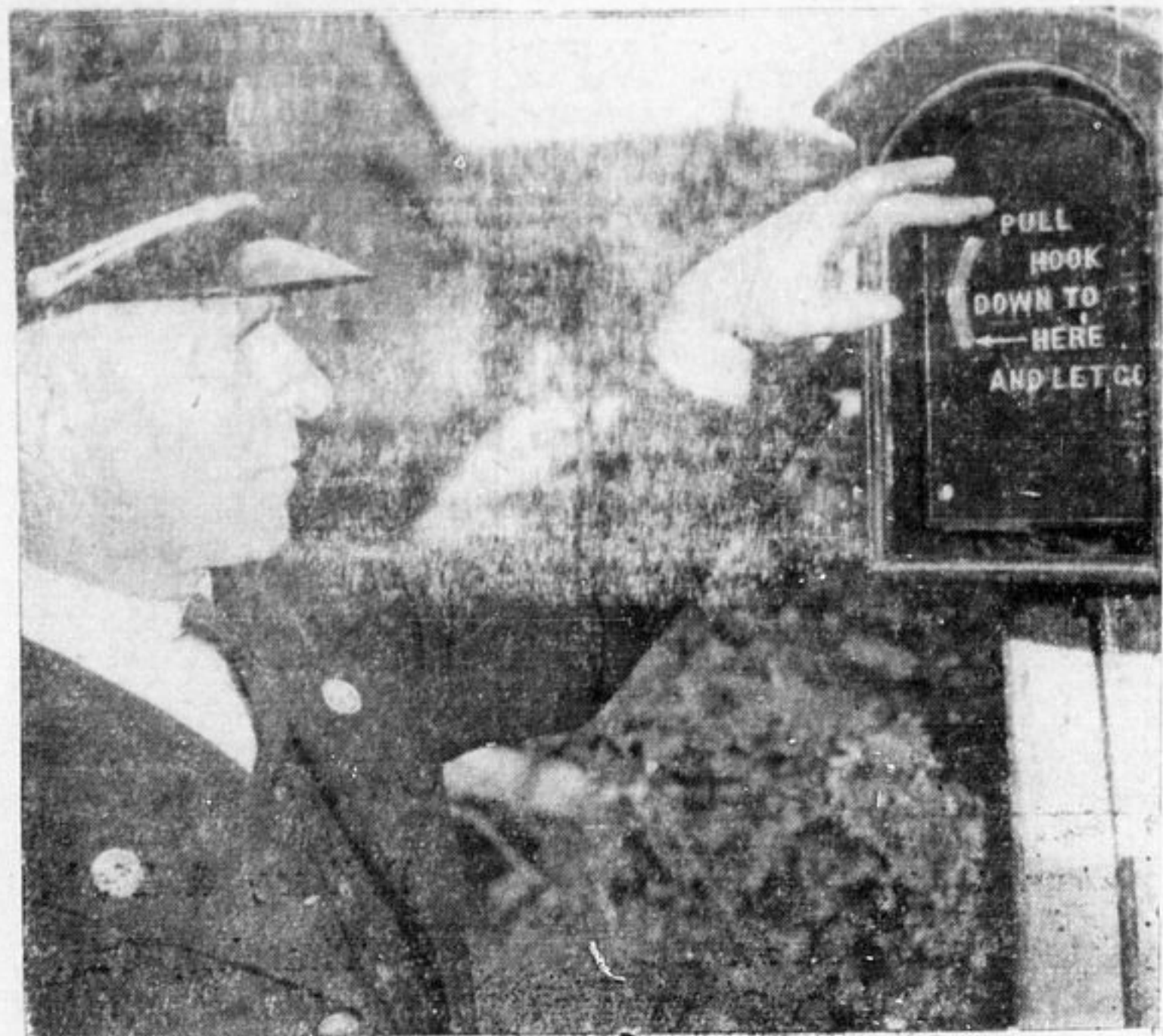
HOW TO RING IN AN ALARM: This is what the interior of the fire box on your neighboring corner looks like. Many persons think that all they have to do is break the glass and turn the knob on the outer door to put in an alarm, Captain Pooley states. Here he shows that the real lever is inside the box. The outside knob merely opens the storm door protecting the unit.
