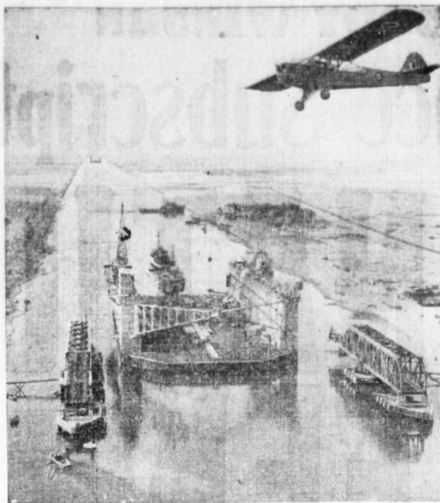
A dock built by the British in Bombay intended for the use of the Royal Navy in Malta, was recently towed there by Admiralty tugs. It is also large (it can accommodate a 50,000 ton ship) that it had to be cut in two for passage through the Suez Canal.
