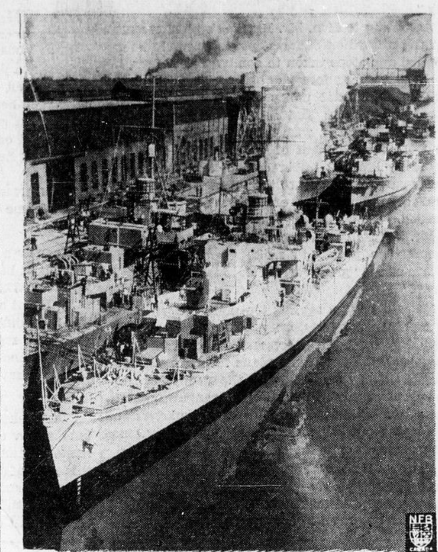
Outstanding achievement in a field where Canadian skill and ingenuity have brought wartime miracles has been the construction of Frigates in Canadian shipyards. The Frigate is one hundred feet longer than the corvette, is faster and more strongly engine, carries heavier armament. The average cost is nearly $1,500,000. Deliveries for 1944 are scheduled at a rate close to one per week, with 44 to be delivered. Above are frigates at fitting dock.
