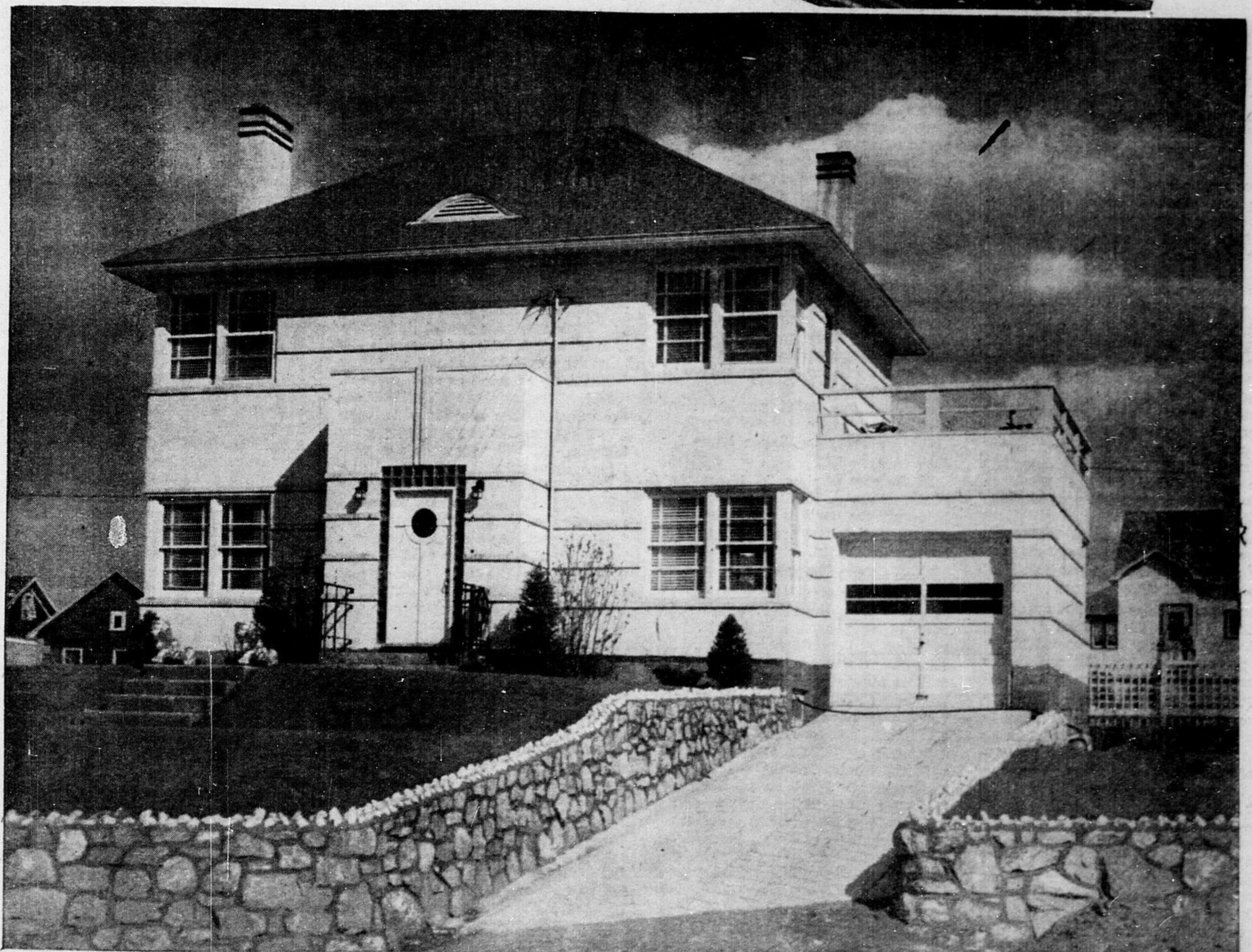
The beautiful home of M. McChesney, 20 Hart Street, built by J. P. Roy, Contractor.
